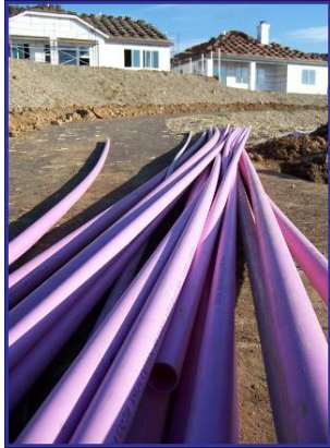
▲ Construction ready to begin
