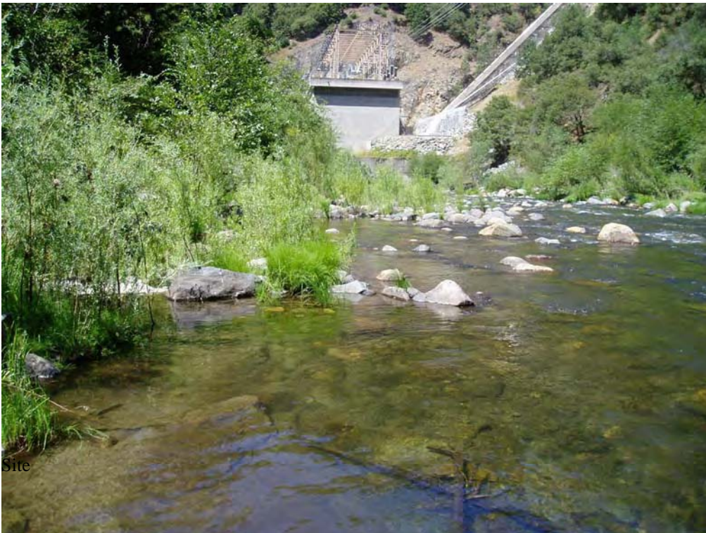
105R-a – SFAR at Akin Powerhouse- top of site looking downstream 105R, August 23, 2005
