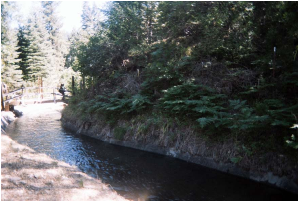
Photo 10: Typical fence upgrade (looking upstream)
