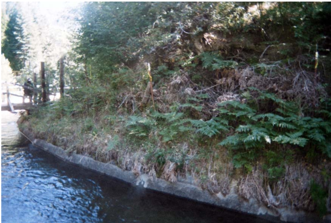
Photo 8: Typical fence upgrade (looking upstream)
