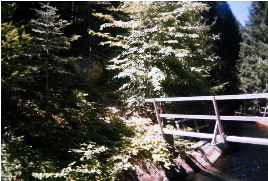
Photo 6: Typical fence relocation
