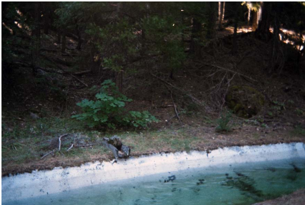
Photo 2: New wildlife crossing approximately 300 feet upstream of No Name Creek
