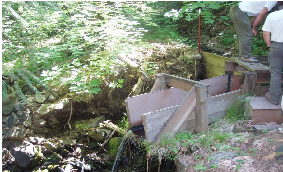
Figure 4. The existing Ogilby Creek diversion and flow bypass structure.
