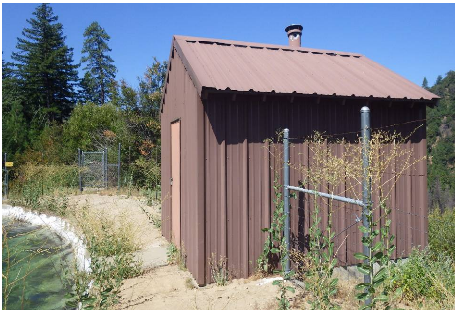
Photo B6 – Warming Shed East of Spillway 7
