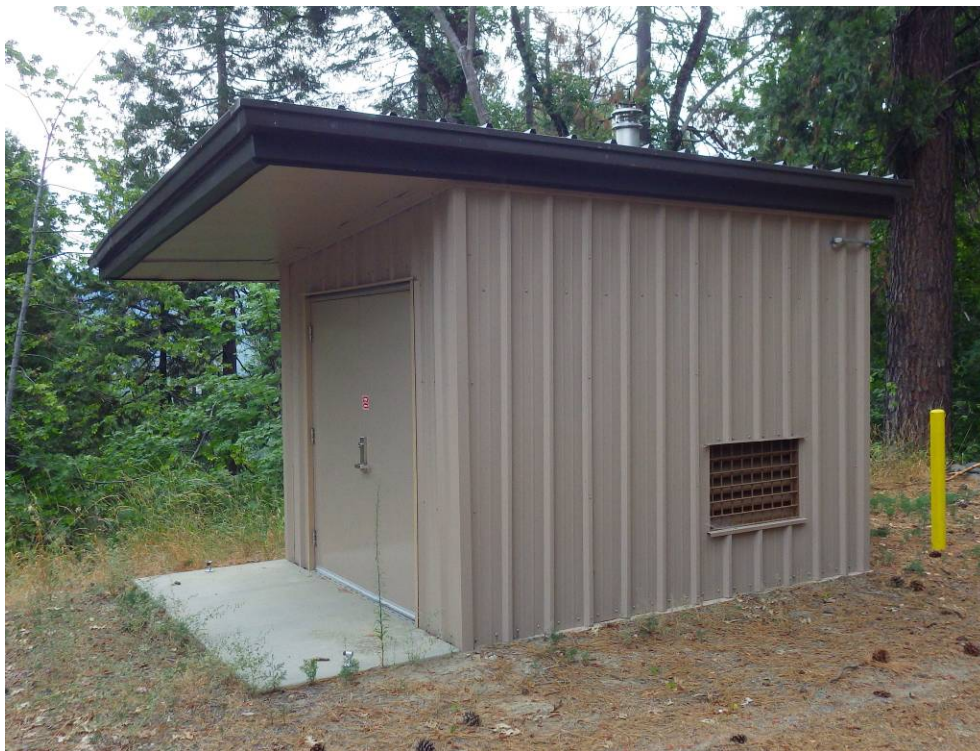
Photo B16a – Spillway 23 Generator House
