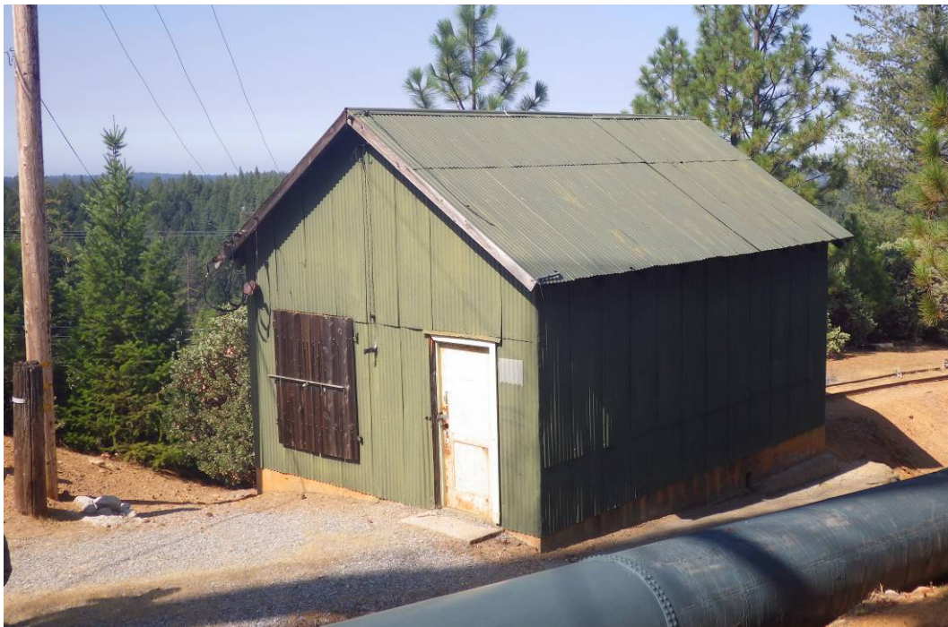
Photo B20 – Winch House Near Surge Chamber
