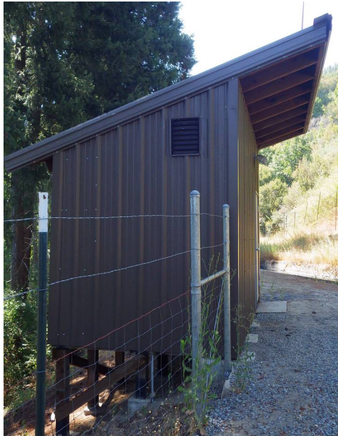
Photo B7 – Spillway 10 Storage Shed (updated)
