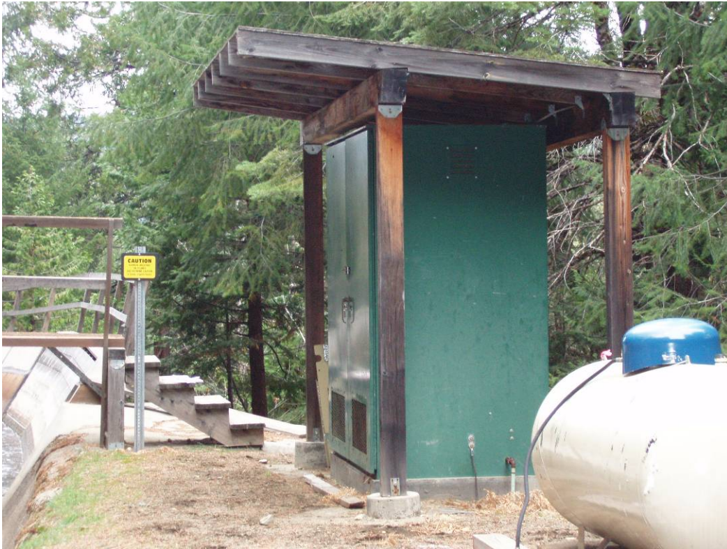
Photo B16 – Spillway 23 Generator House (Removed in 2014)
