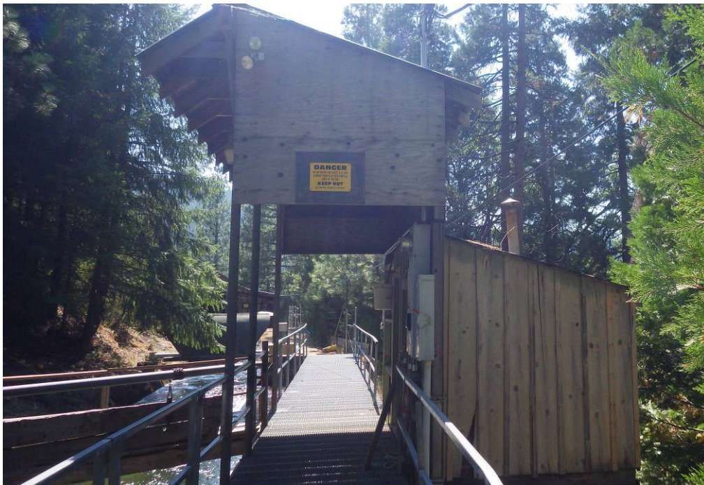
Photo B13 – Spillway 20 Warming Shed
