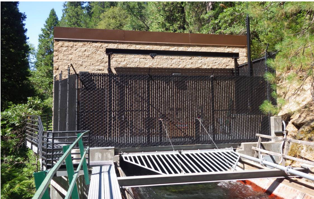
Photo B11 – Spillway 20
