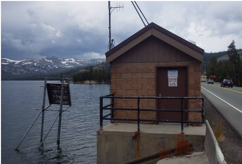
Photo B5 – Caples Control Room
