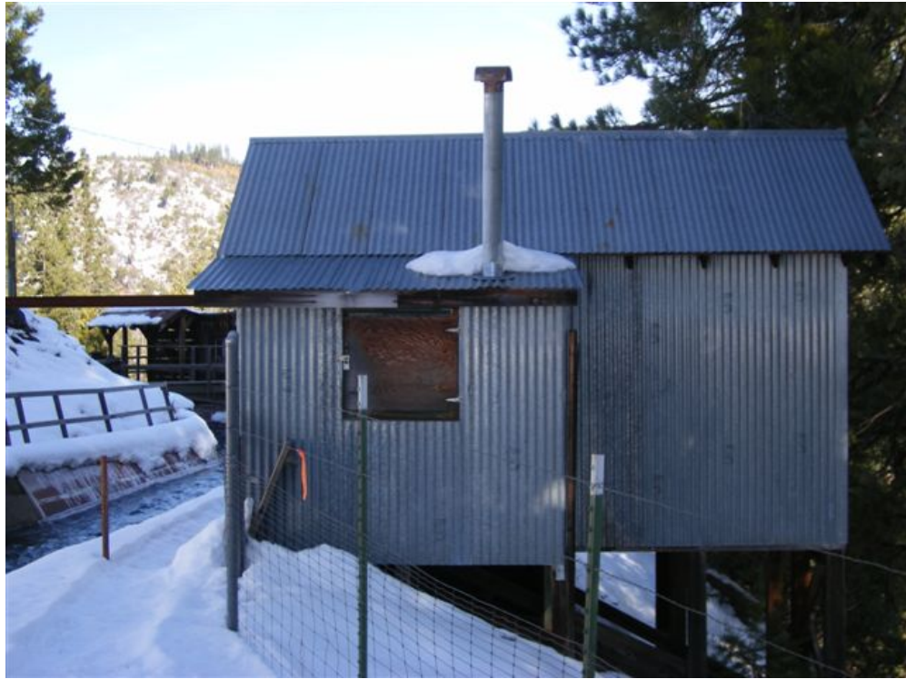
Photo B7 – Spillway 10 Boat House (Removed in 2011)
