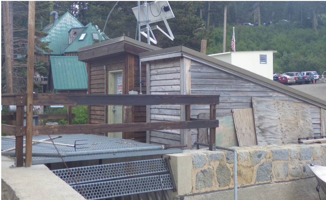
Photo B1 – Echo Lake Control Room (updated)
