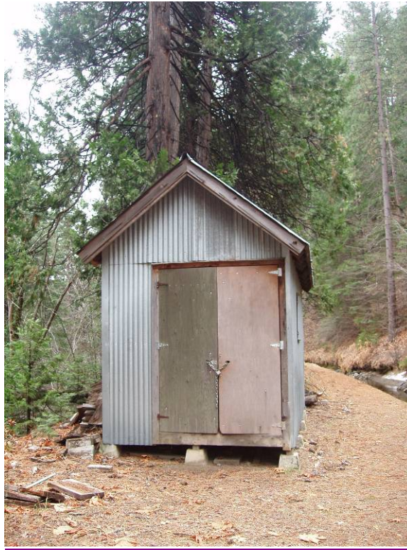
Photo B17 – Rock Crusher Storage Shed (Removed in 2013)
