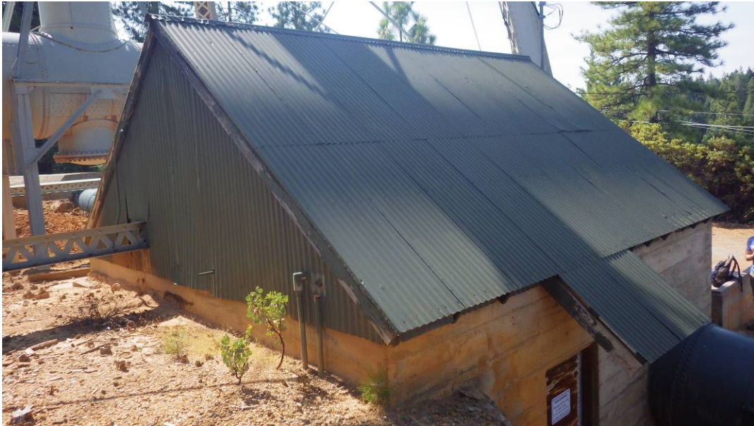
Photo B19 – Lower Butterfly Valve House
