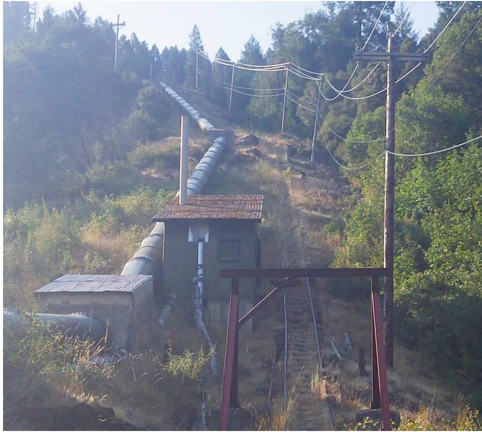
Photo B21 – Water Tank Shed
