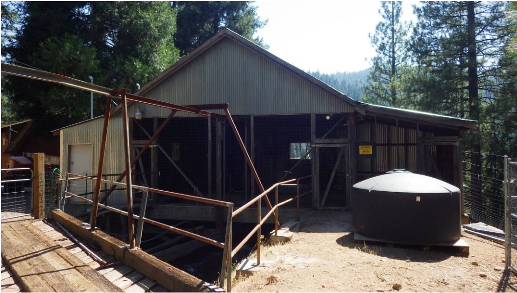
Photo B14 – Plum Creek Siphon House
