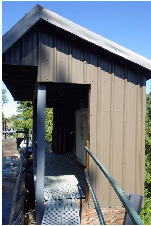
Photo B8 – Spillway 10 Building (updated)
