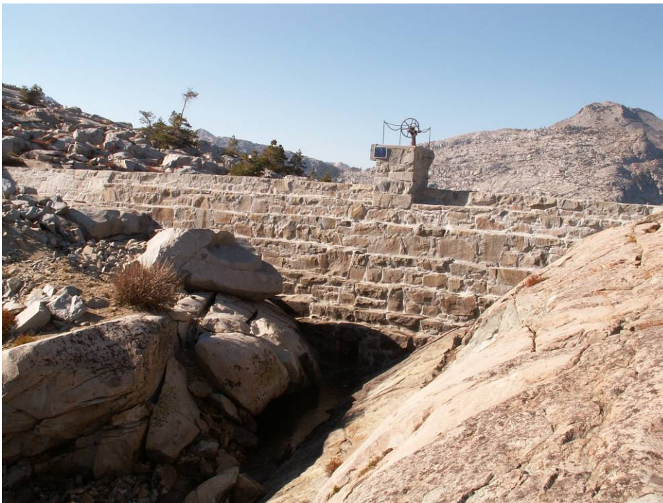
Photograph B-2. Lake Aloha Main Dam.
