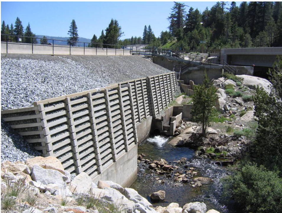
Photograph B-22. Silver Lake Dam (back) and Fish Ladder.
