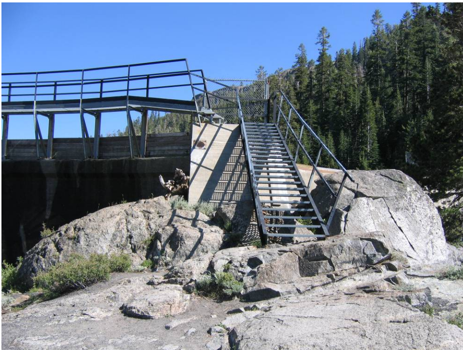
Photograph B-14. Caples Lake Auxiliary Dam and Metal Staircase/Walkway.
