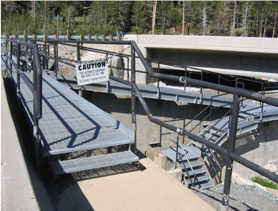
Photograph B-23. Silver Lake Dam Metal Walkway and Railings.
