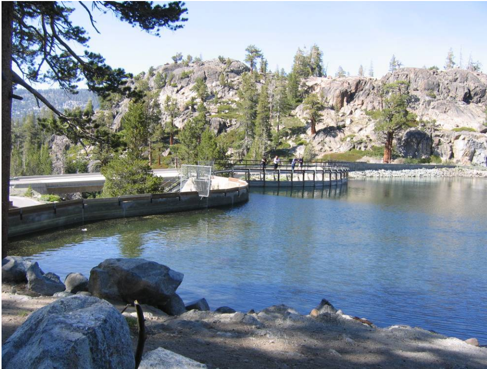
Photograph B-13. Caples Lake Auxiliary Dam.
