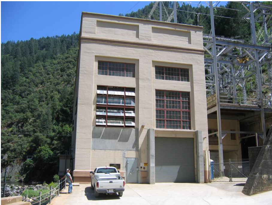
Photograph B-32. Akin (El Dorado) Powerhouse.
