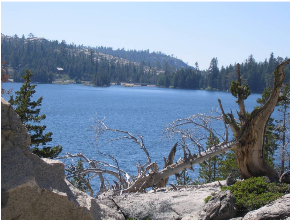
Photograph B-24. Silver Lake Dam (Viewed from Eastern Shoreline).
