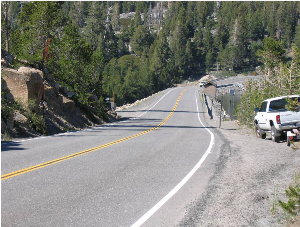
Photograph B-11. Caples Lake Main Dam and State Highway 88.
