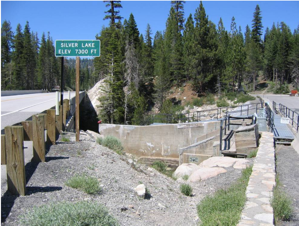
Photograph B-21. Silver Lake Dam and State Highway 88.
