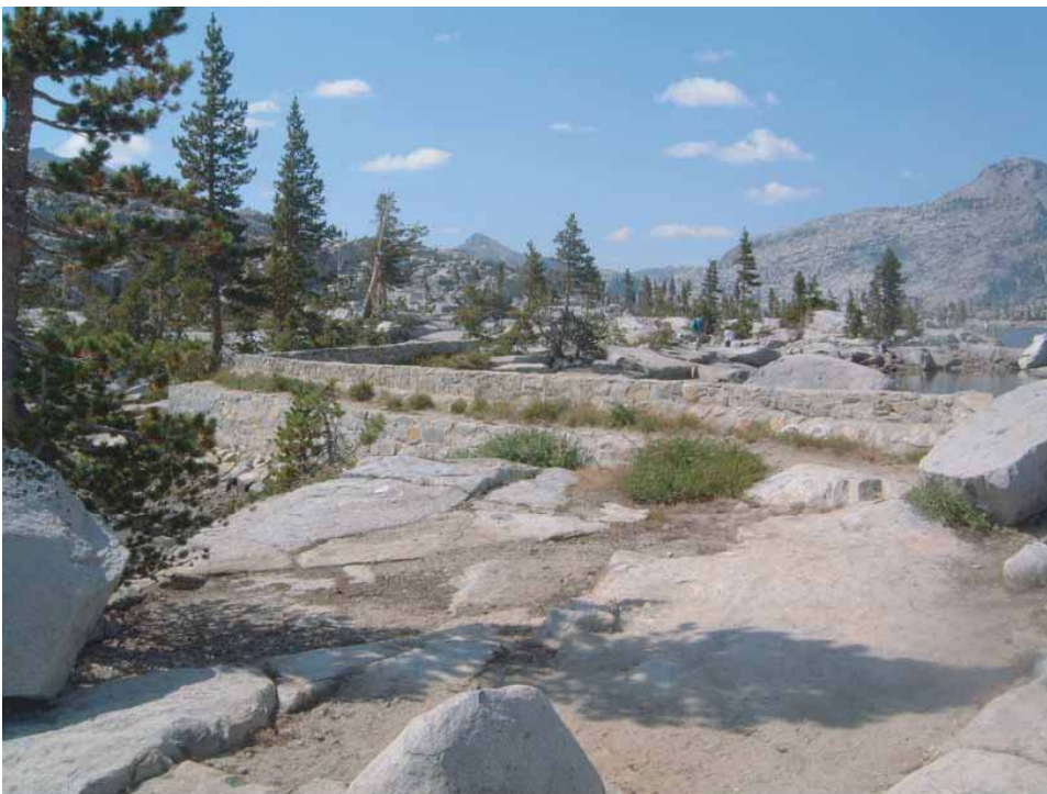
Photograph B-4. Lake Aloha Auxiliary Dam.
