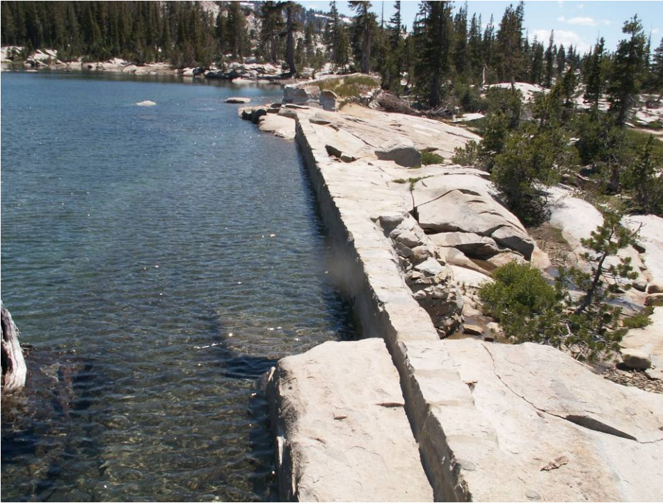
Photograph B-3. Lake Aloha Spillway.
