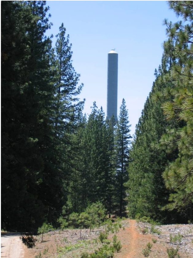
Photograph B-31. El Dorado Surge Tank.
