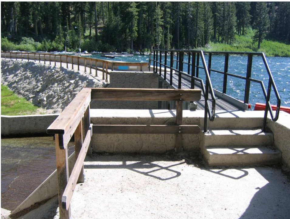
Photograph B-8. Echo Lake Dam and Metal Walkway over Spillway.
