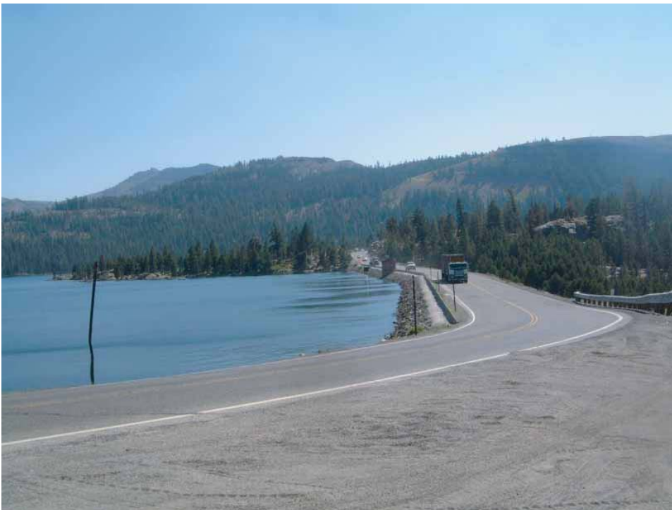
Photograph B-10. Caples Lake Main Dam and State Highway 88.
