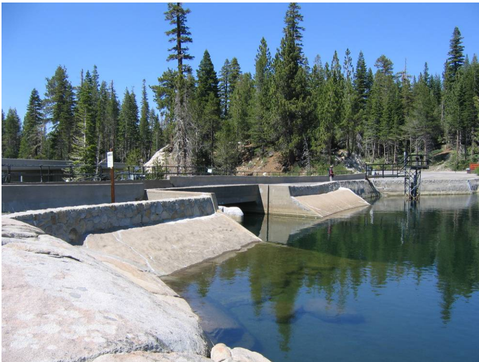
Photograph B-18. Silver Lake Dam and Spillway.
