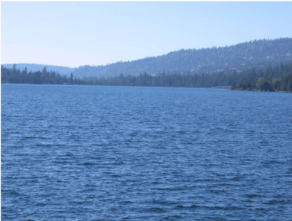
Photograph B-12. Caples Lake Main Dam (Viewed from Woods Creek Lake Access).
