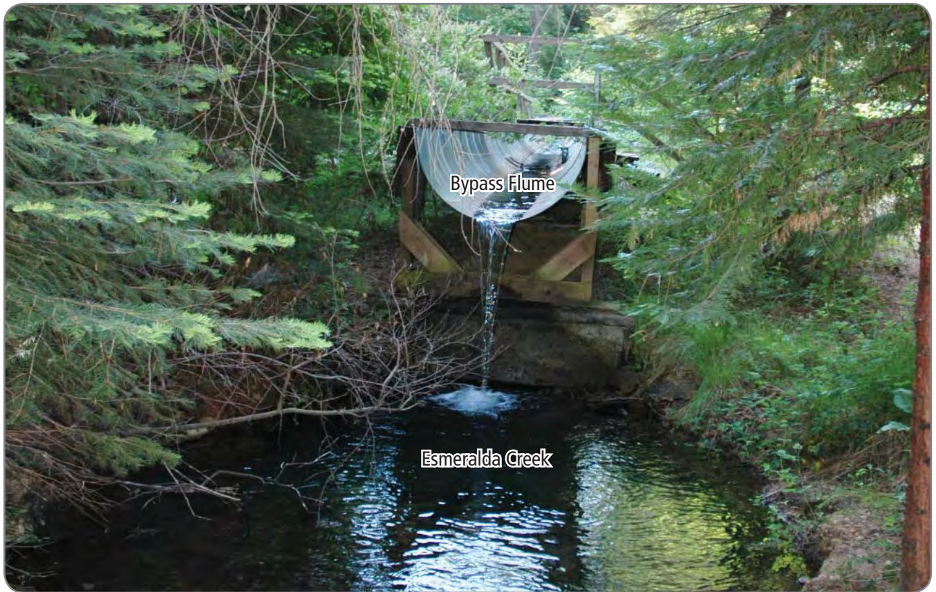
FIGURE 2a: Photo (top) of the El Dorado Canal, Esmeralda Creek diversion and bypass flume (looking upstream). Bypass flume outlet (bottom).
