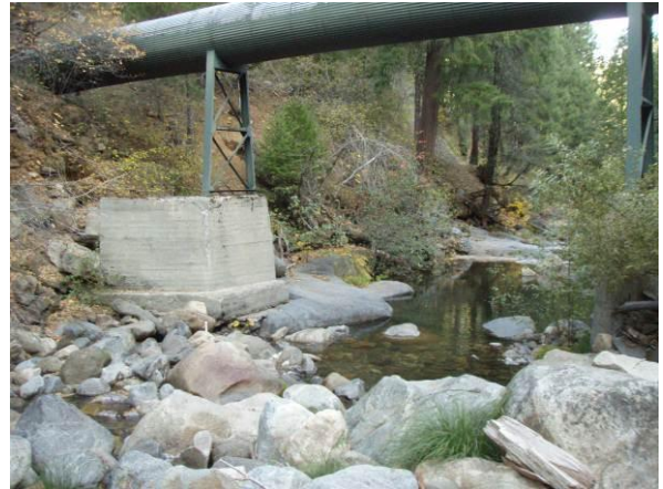
FIGURE AR-B1-4. Looking downstream from the middle transect (F) at Site AR-B1
