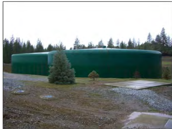
Photo 9 – Tanks and Pressure Reducing Station at Reservoir 7
