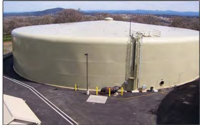
Photo 3 – One of Bass Lake Tanks
