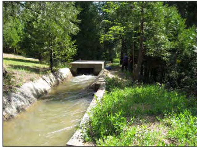
Photo 5 – Outlet Structure at Buffalo Hill
