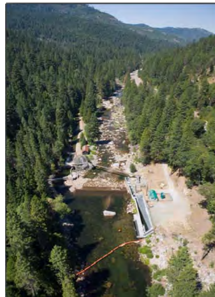
Photo 11 – El Dorado Canal Diversion on South Fork American River near Kyburz
