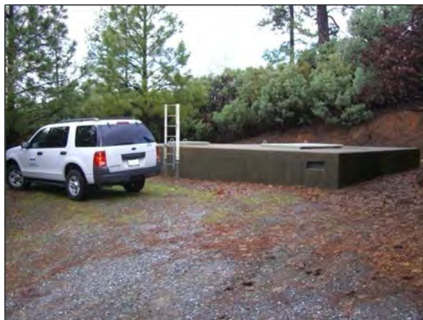
Photo 2 – El Dorado Main 2 Pressure Reducing Station No. 3 west of Reservoir 3
