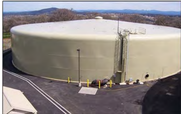
Photo 3 – One of Bass Lake Tanks
