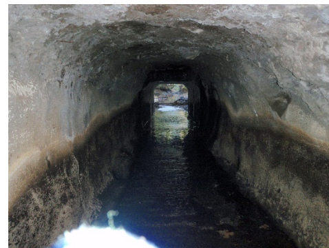
14-mile tunnel inside looking downstream
