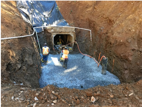
2018 14-mile Tunnel-box culvert connection foundation preparation
