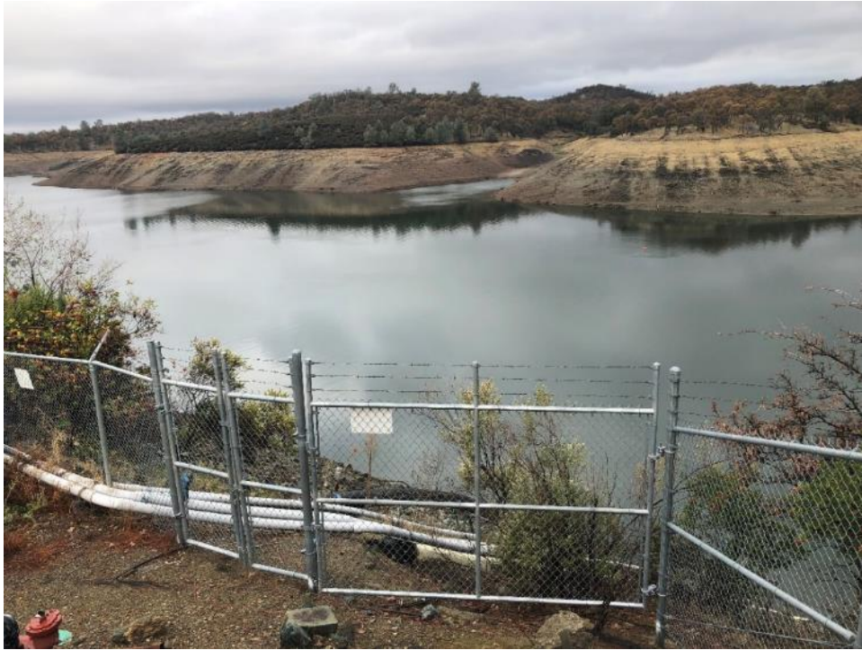
View of Folsom Lake and existing pipes.
