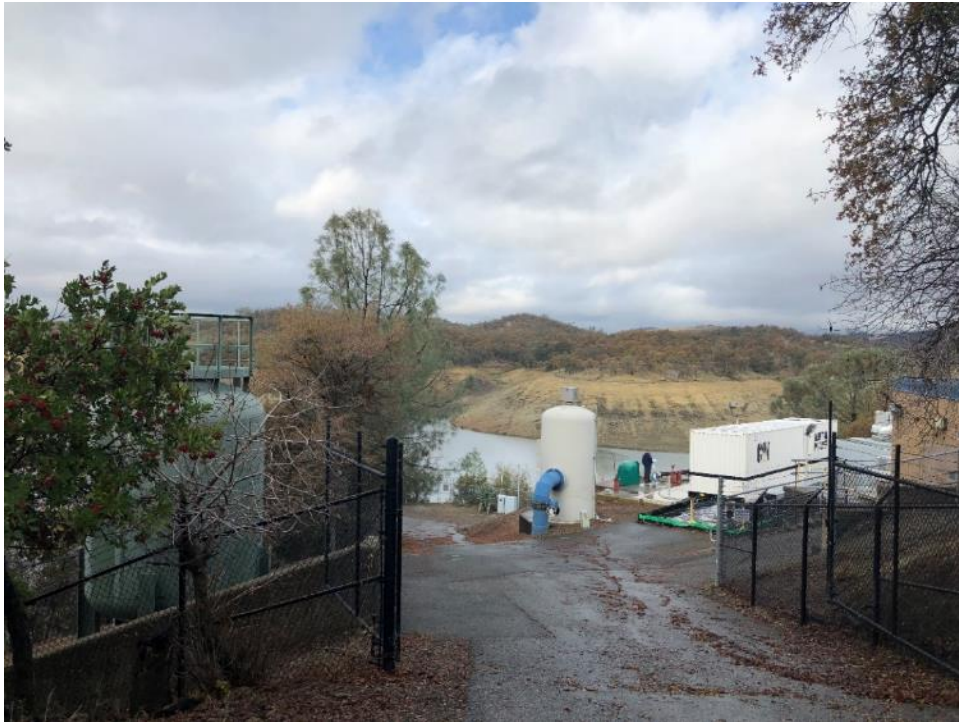
View of existing facilities within developed area of project site.
