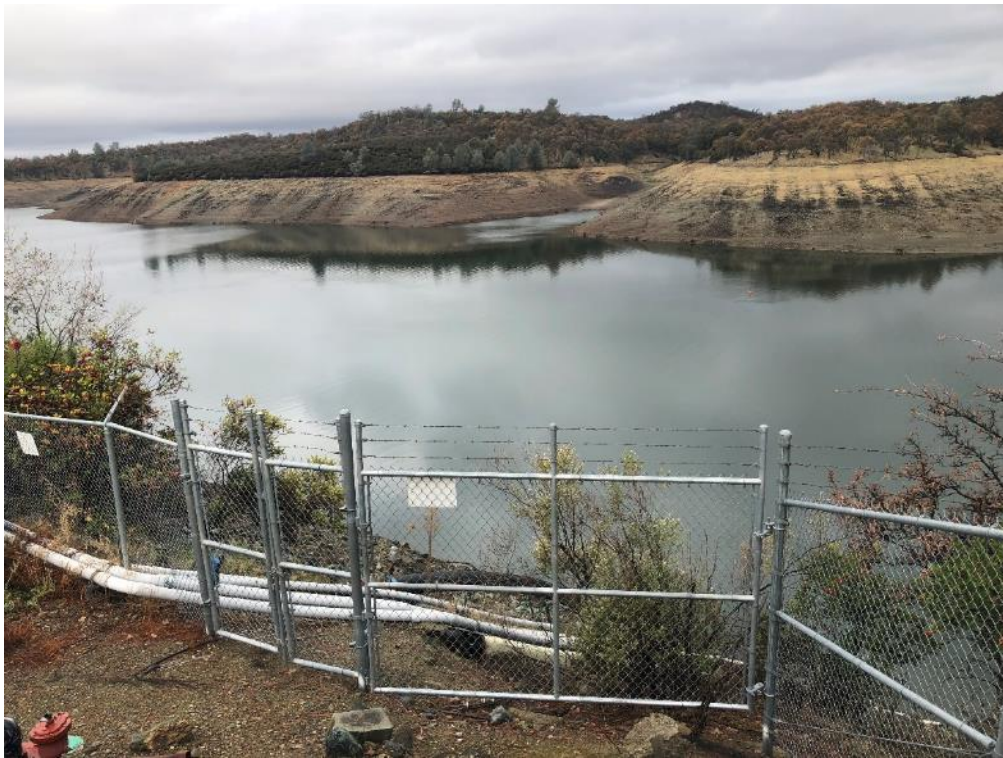
View of Folsom Lake and existing pipes.
