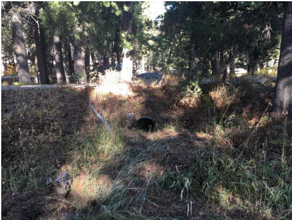
View of existing culvert crossing the campground roadway.
