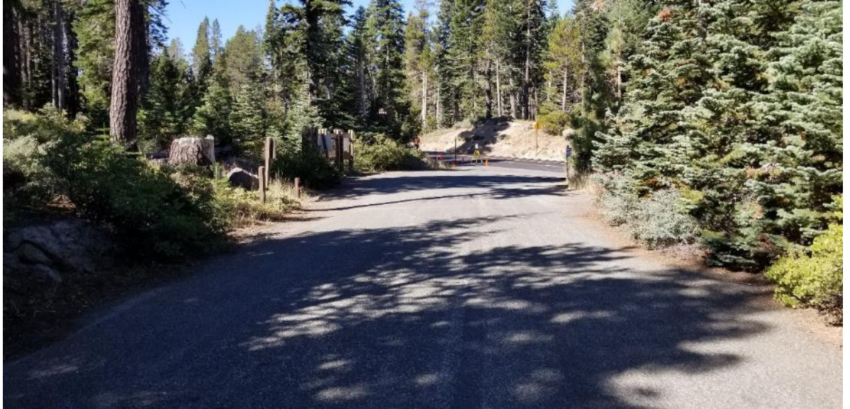
View of Silver Lake Campground water supply alignment at entrance to campground loop road.
