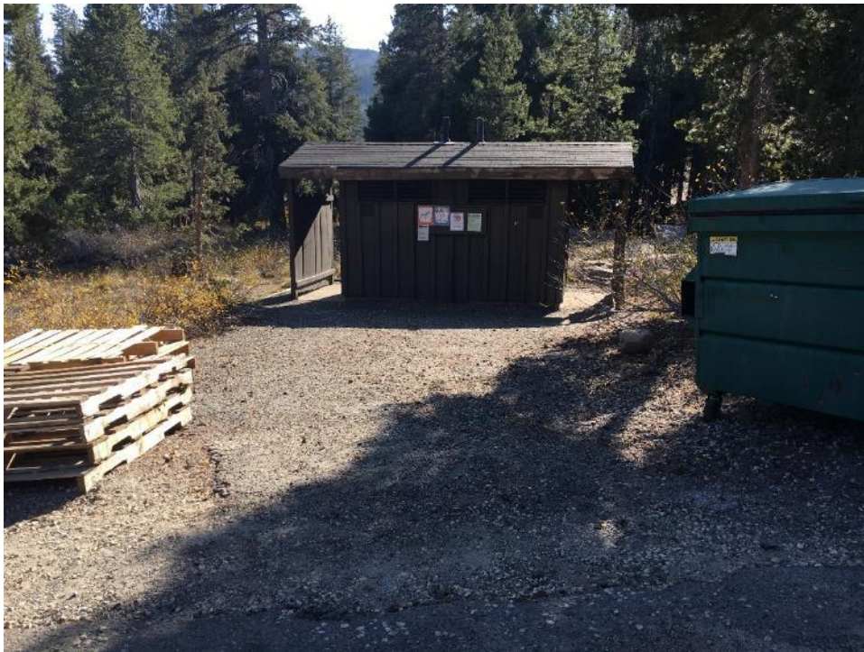
View of existing vault toilet facility and waste disposal access.
