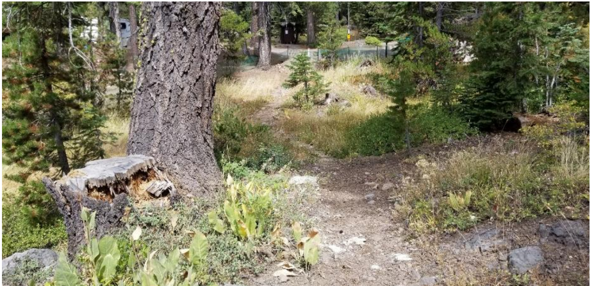
View along Silver Lake Campground water supply pipeline alignment.
