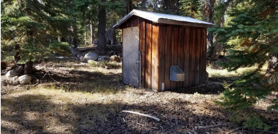
View of existing well enclosure structure.
