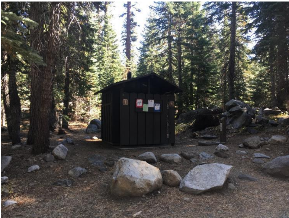
View of existing vault toilet facility.
