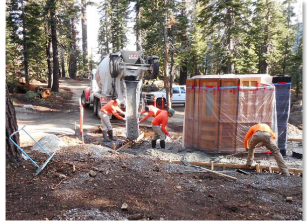
Placing Concrete at Caples Lake West Campground
