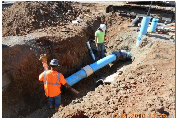
Installing 12" C-900 and HD Coupler
