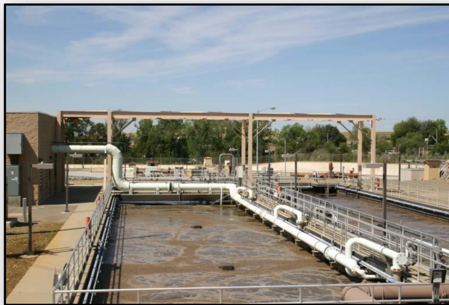
El Dorado Hills wastewater treatment plant (EDHWWTP)
