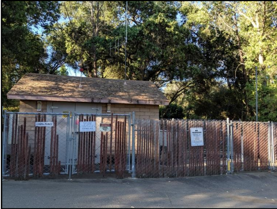
Sewer lift station upgrades $3.7 Million over 5 years
