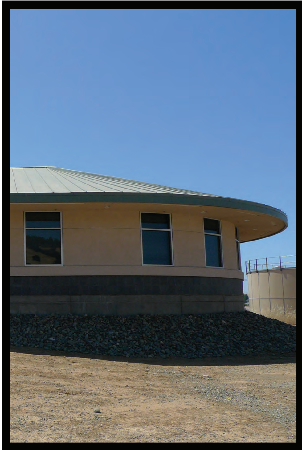
The new El Dorado Hills Wastewater Treatment Plant operations building. This building is part of the two-year, $54.7 million regulatory upgrade and capacity expansion at the plant.
