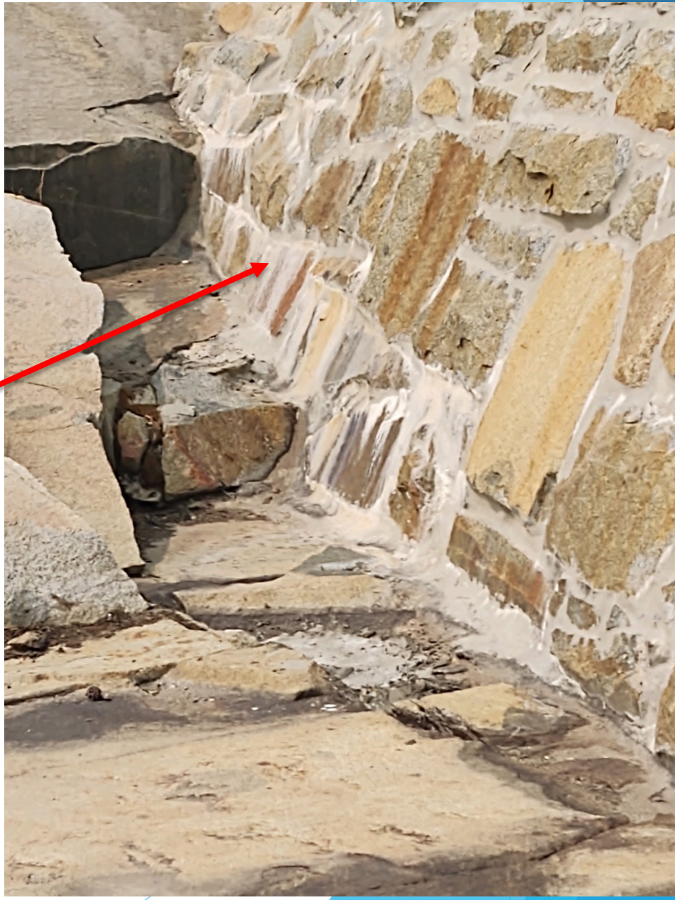
Mortar Repairs to Dams 6 & 7
