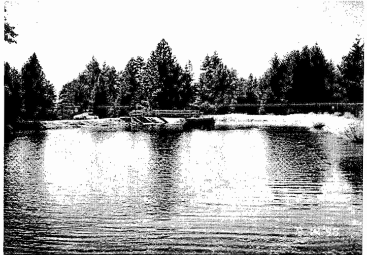
Reservoir A prior to construction.
