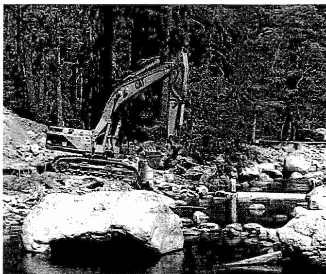
The Diversion Dam, part of Project 184, under construction.
