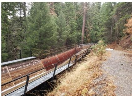
**Flume 45 Abutment Section Replacement:** This section of Flume 45 is an elevated wood flume approximately 100 feet in length and was last replaced in 1945. This portion of the flume was constructed to span a section of the historic rock bench that had previously failed. The replacement of this section of flume is expected to occur during the scheduled canal outage in 2022. This project will only address the abutment section. The remainder of Flume 45 will be addressed in future CIPs.
