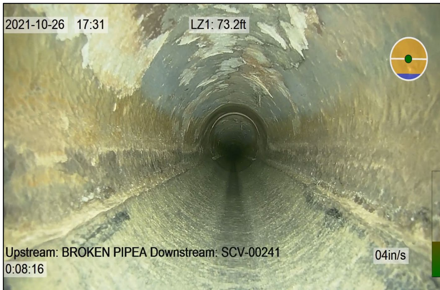
Corroded Pipe
