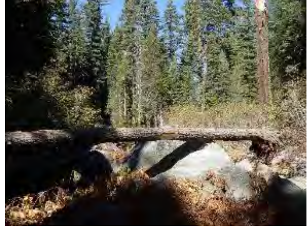
FIGURE SH-B1-2. Looking downstream from the bottom transect (A) at Site SH-B1 (from 2017)
