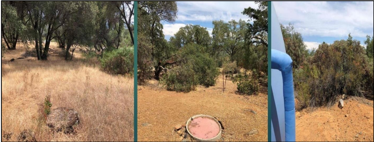
Figure 2-5. Typical Segment of Diamond Springs Main Right-of-way
