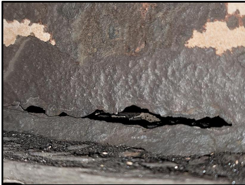
**Perforation at webbing/lower flange, post blast.**
