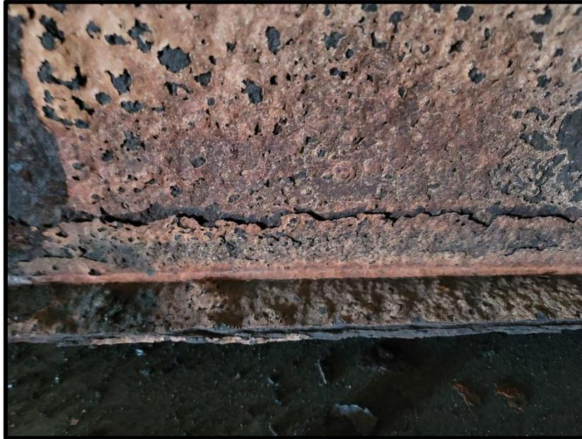
**Stratified Corrosion at webbing on rafter.**
