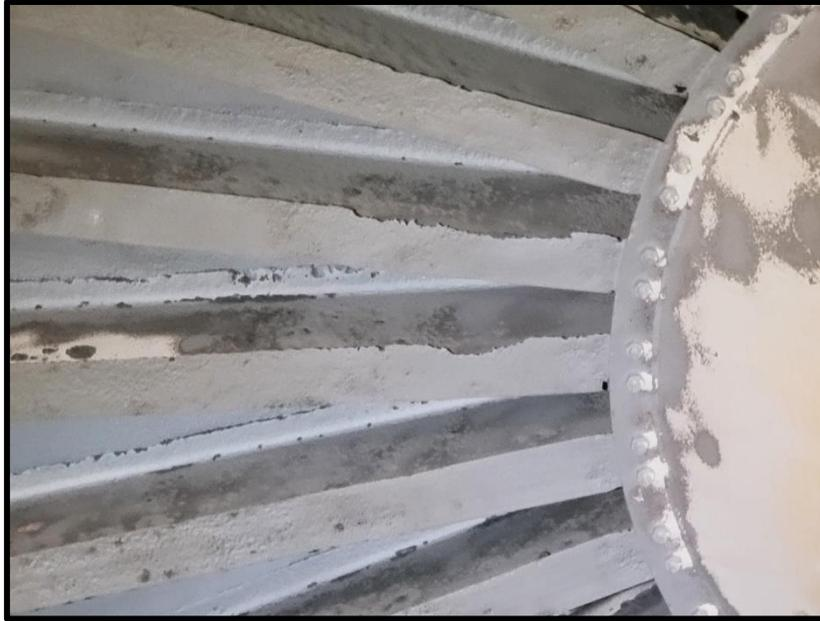
**Massive metal loss @ center rafters and dollar plate.**
