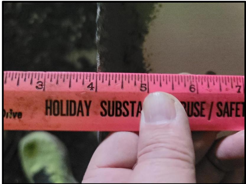
Outer rafter flange after removing corrosion 1/16 = UNSAT.
