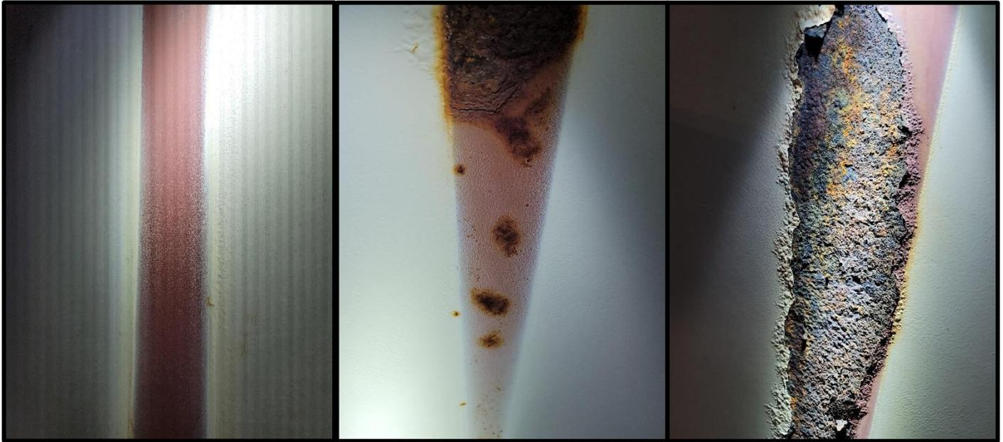
Outer Pass Roof Plate @ Rafter Interface, difference between contact and non-contact points varied in conditions from full intact primer to heavy stratification with clear signs of heavy metal loss, including perforation (identified on good side of tank).
