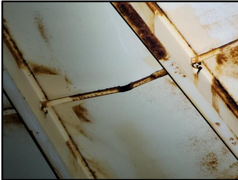
Heavy corrosion and metal loss at Seismic Straps.
