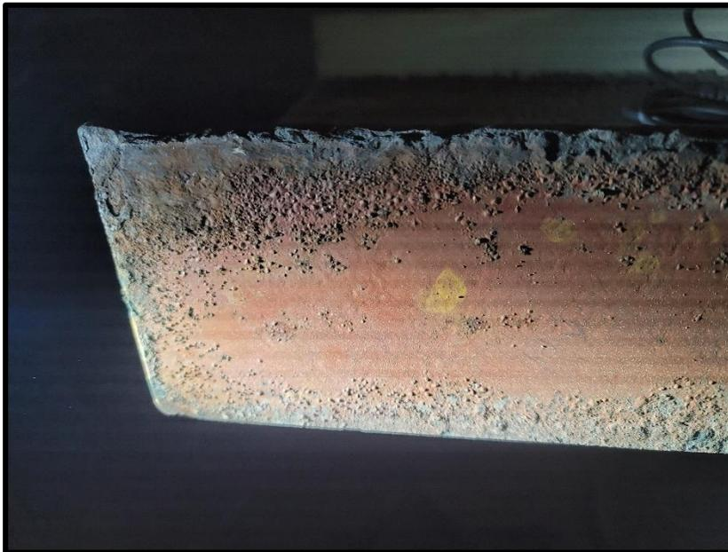
**Outer rafter showing only shop prime applied, also blast media inclusions visible.**
