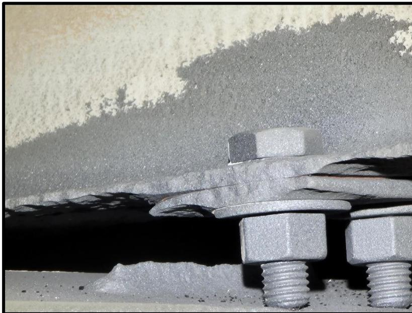
**Outer rafter/girder interface, rafter clip disintegrated due to corrosion.**
