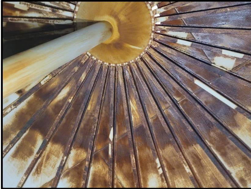
**Heavy corrosion visible at center rafter @ dollar plate.**
