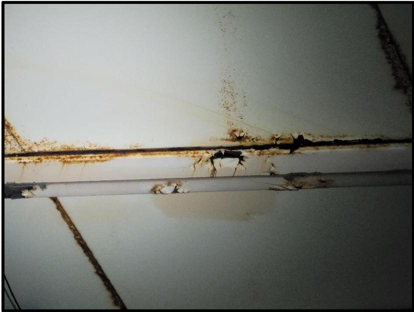
**Main concern on outer pass is the contact points at roof/rafter interface.**
