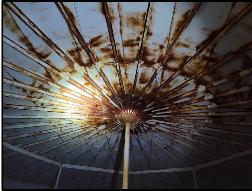
General overall condition, Intact coating, Surface corrosion, Heavy corrosion at center.
