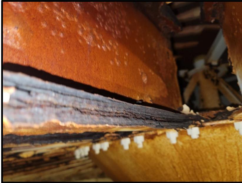
**Heavily stratified flanges both upper and lower @ Center Rafters.**
