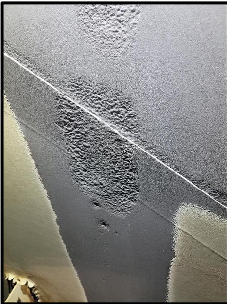
Roof corrosion on 3/16 plate.
