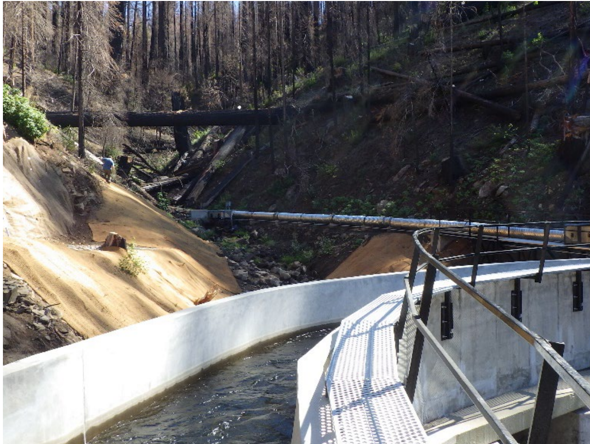
Flume 30 reconstructed as a wildfire resistant concrete canal.
