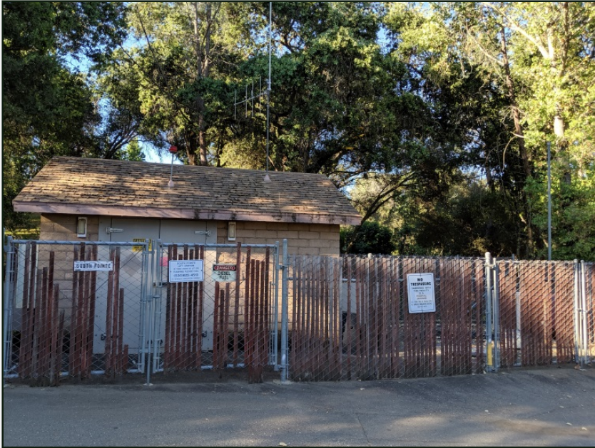
SEWER LIFT STATION UPGRADES $9 MILLION
