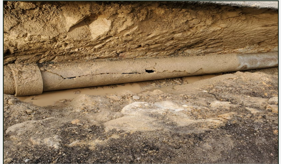
PIPELINE REPLACEMENT $20 MILLION
