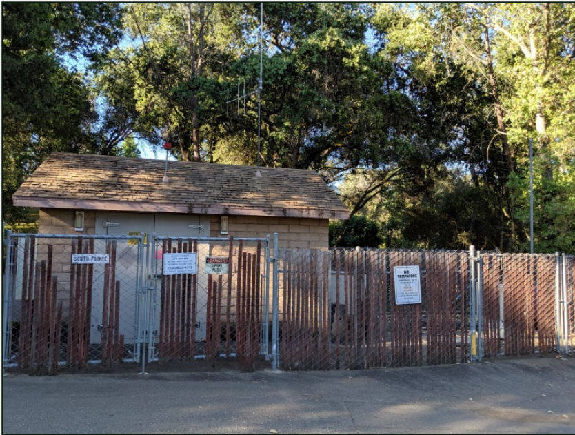
SEWER LIFT STATION UPGRADES $9 MILLION
