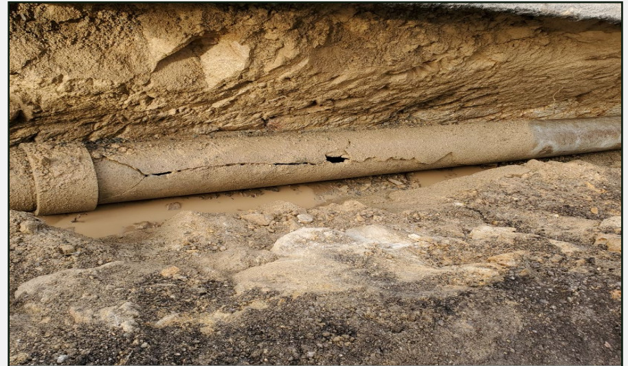
PIPELINE REPLACEMENT $20 MILLION
