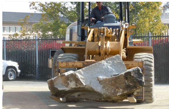
Blasted Piece of Granite Rock for the SJWD 72" Pipeline Trench
