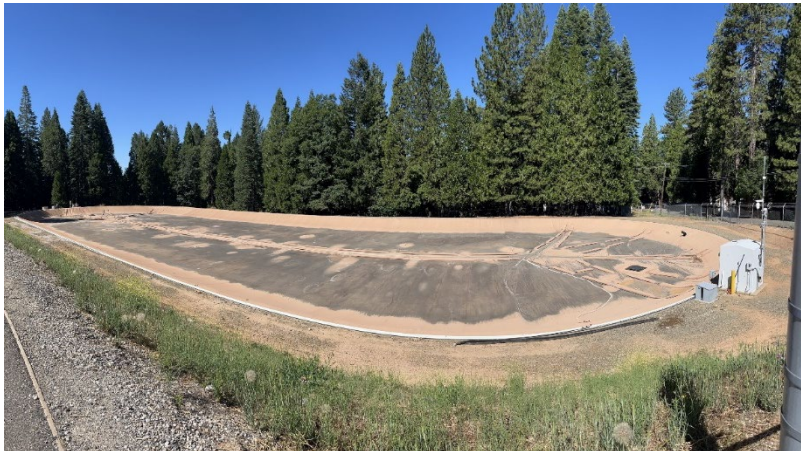
Reservoir 1 floating cover
