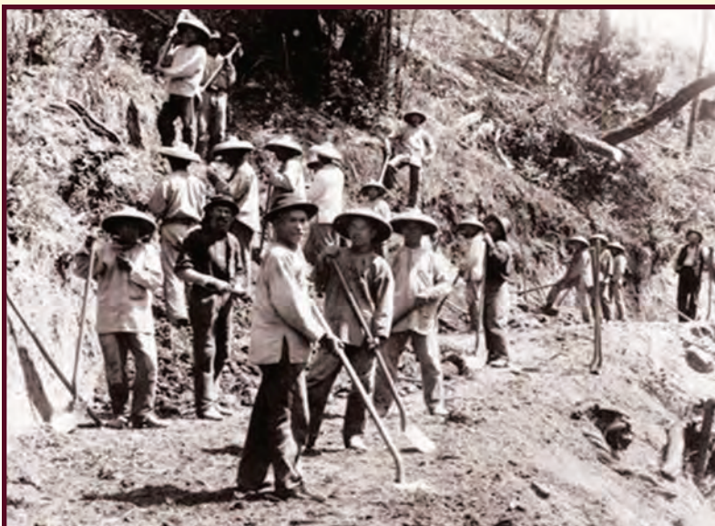
Two major eras of ditch and canal building occurred in El Dorado County. The first (1852 – 1858) provided water for sluicing and hydraulic mining once the easy gold diggings in streams paid out. The second phase (1867 – 1880) helped for a short time to revive gold mining as one response to the nationwide depression of 1873. Agriculture and towns also benefitted from the canals.
