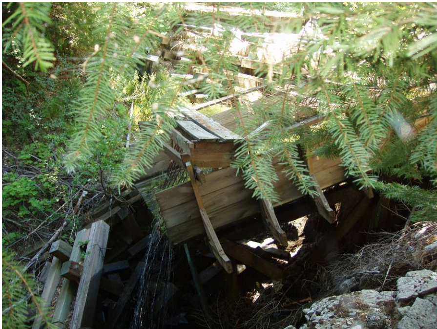
Photo B2 – Wooden Box Outlet at Spillway 3
