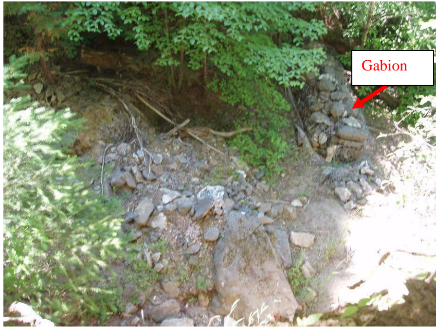
Photo B5 – Spillway 20 A/B Gabion (sediment trap)
