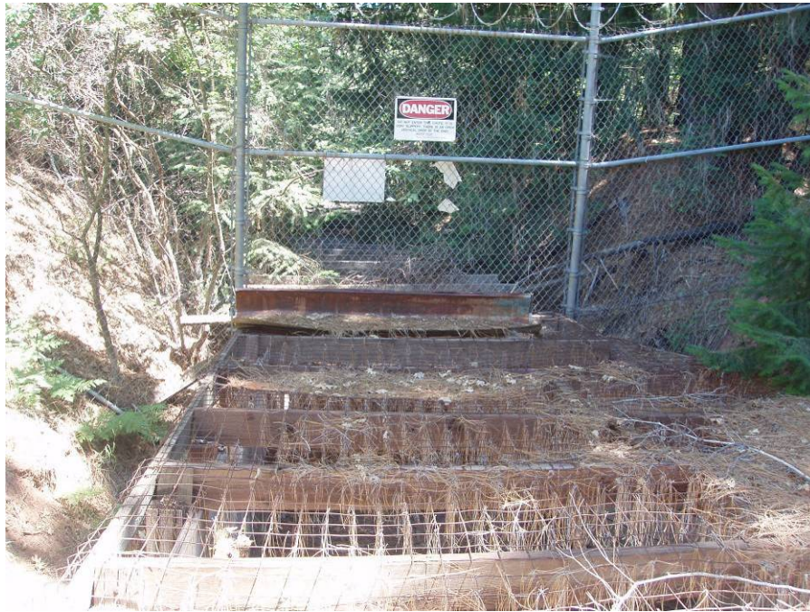
Photo B11 – Spillway 47c Wooden Spillway Outlet
