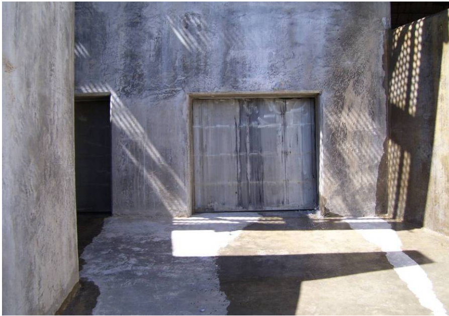
Photo A3 – Example Sluice Gate
