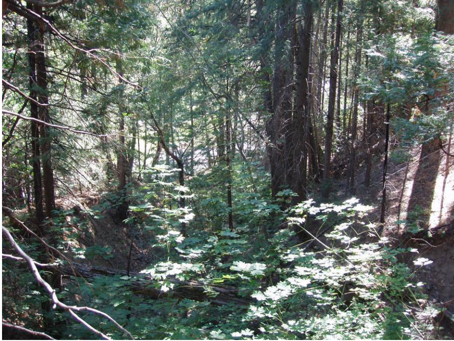
Photo B1 – Spillway 3 Channel
