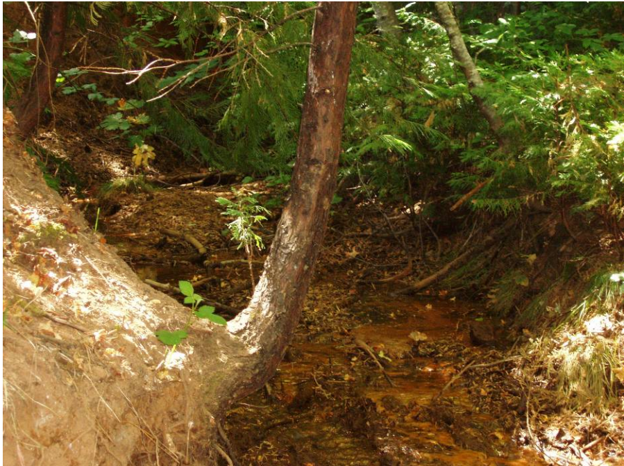
Photo B10 – Spillway 37 Downstream Channel near Freshpond
