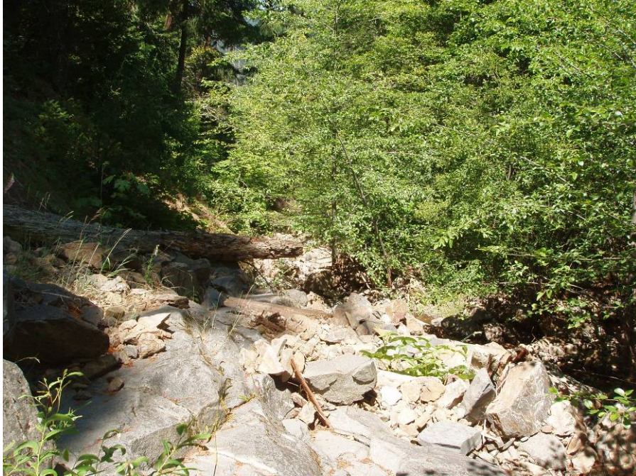
Photo B7 – Spillway 27 Channel
