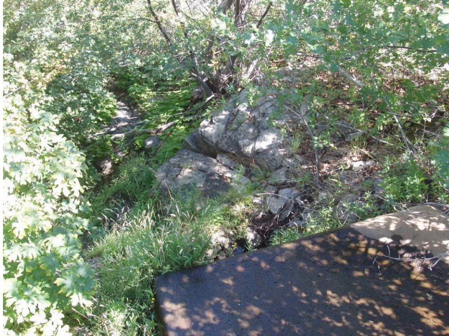
Photo B3 – Spillway 11 Outlet and Channel
