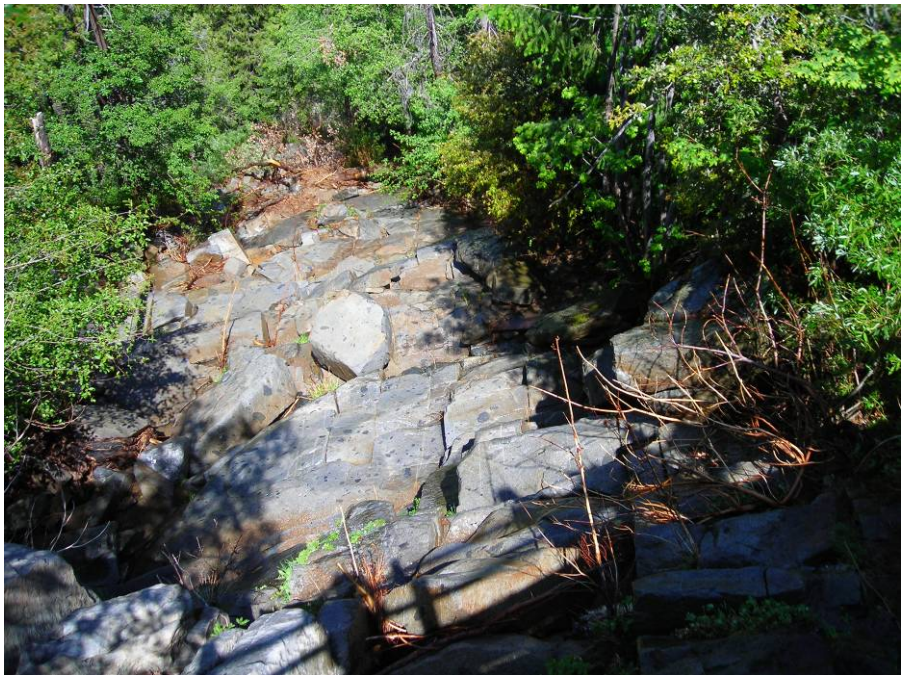
Photo A6 – Example Rock-Lined Spill Channel
