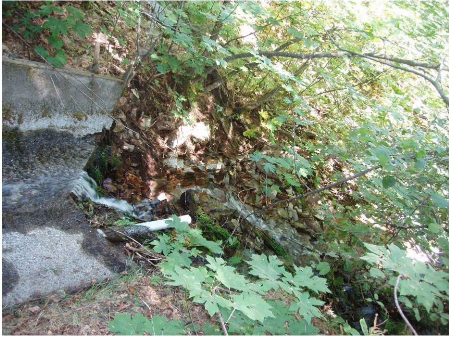
Photo B9 – Spillway 33 Outlet and Channel
