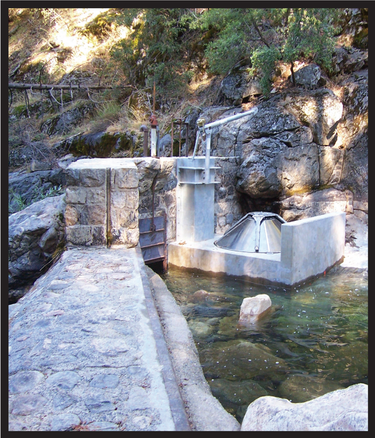
Alder Creek Diversion fish screen installation as required to meet a Project 184 license condition.
