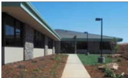
The new Suncoast Professional Center is the first building in El Dorado Hills Business Park to use recycled water for landscape irrigation.
