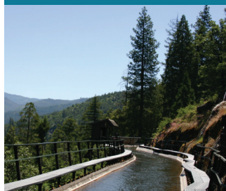
Flume 13 /Spillway 10—water for customers and energy
