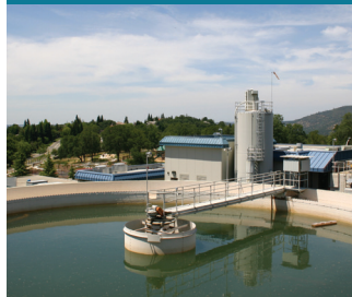
El Dorado Hills Water Treatment Plant
