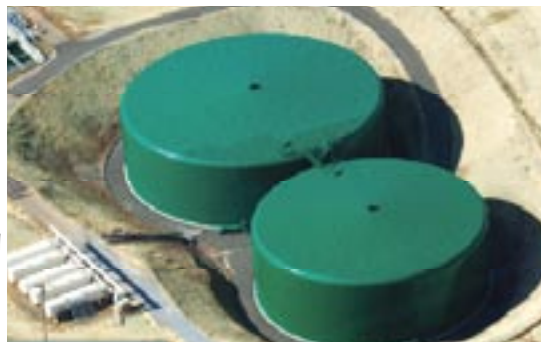
Completed steel tanks at Reservoir 7 in Diamond Springs
