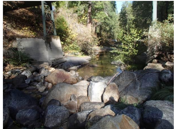
FIGURE AR-B1-4. Looking downstream from the middle transect (F) at Site AR-B1
