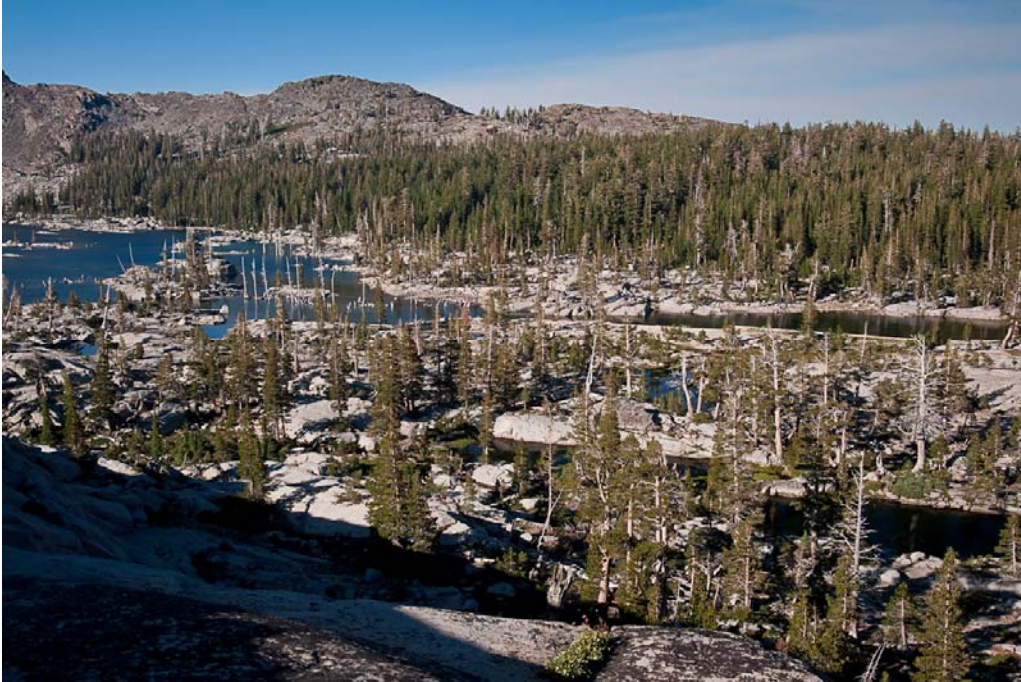
Photo 37. Overview of Auxiliary Spillway: Ponds below dams. Pond E is the nearest pond. 8/04/10
