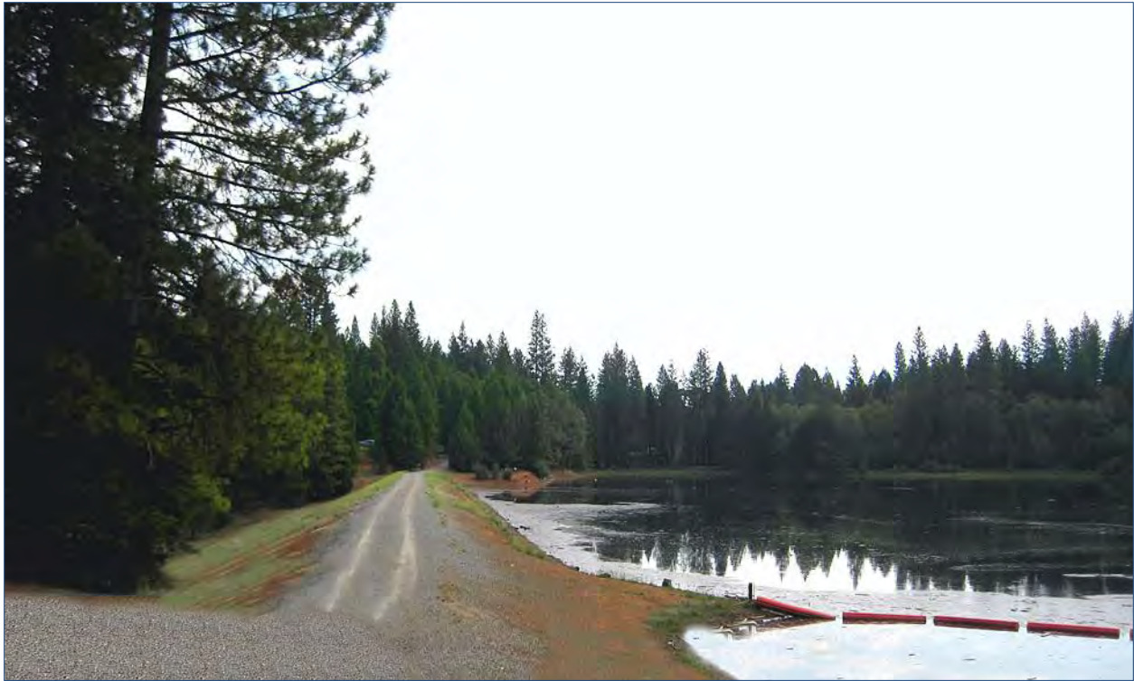
Existing view from Viewpoint 8 (view from dam near Main Ditch Intake). The fence around the spillway has been digitally removed to allow a more accurate comparison to the photosimulated perspective. The fence would be retained or replaced as part of the Project.
