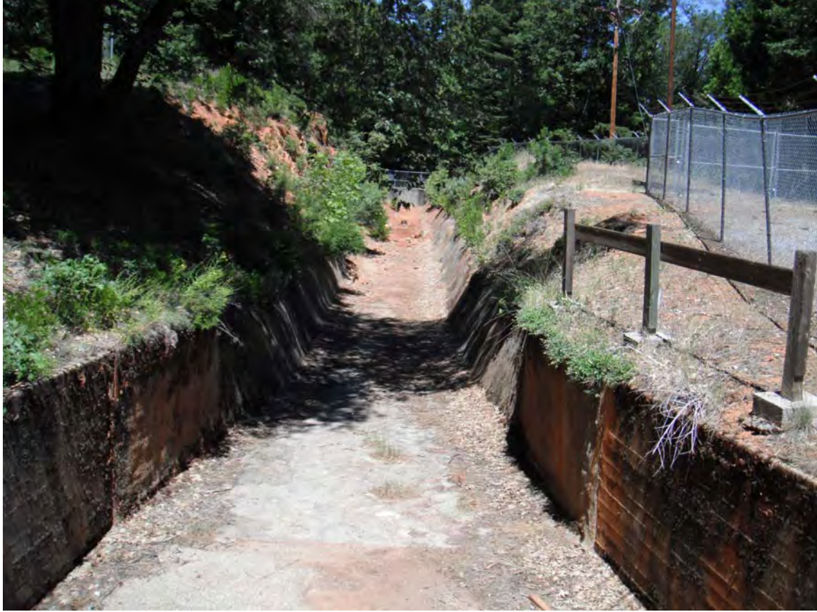
The emergency spillway channel at southwestern corner of Forebay.
