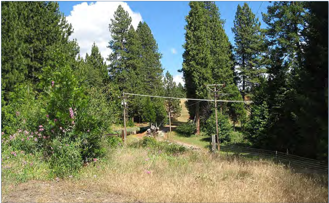
Viewpoint 6: View from Forebay Road where it crosses the penstock, looking east toward the dam
