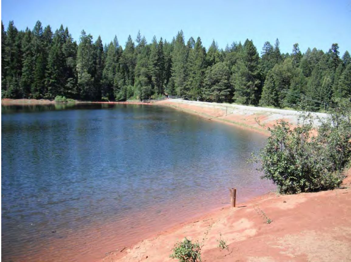
Looking southwest along Forebay dam shore showing bare ground and frequently used walking trail along top of dam.
