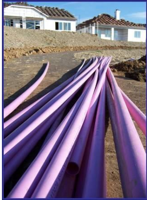
▲ Construction ready to begin
