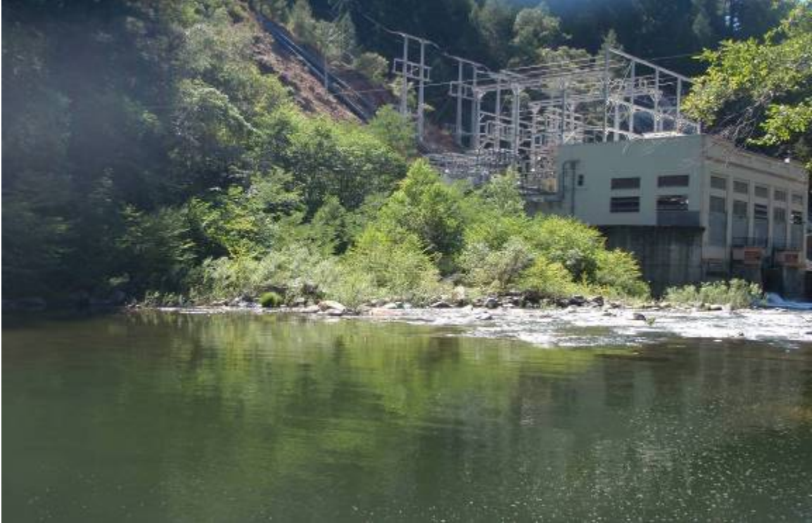
Photo 3. Site 105c – SFAR at Akin Powerhouse, view from the right bank of the SFAR, July 27, 2011.
