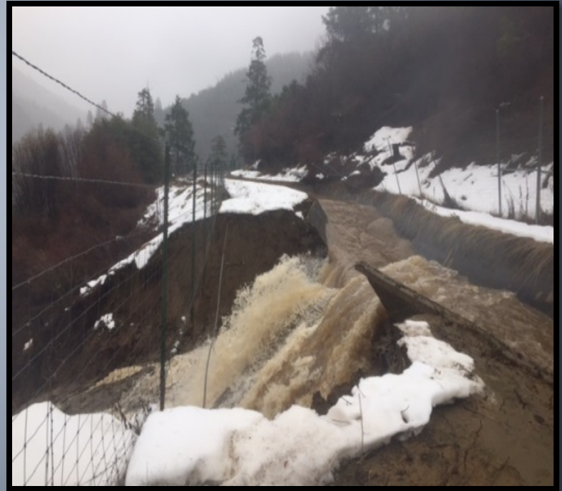
Canal section below Flume 10
