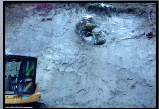
Flume 2A crews cabled loose boulders on 1/6/17
