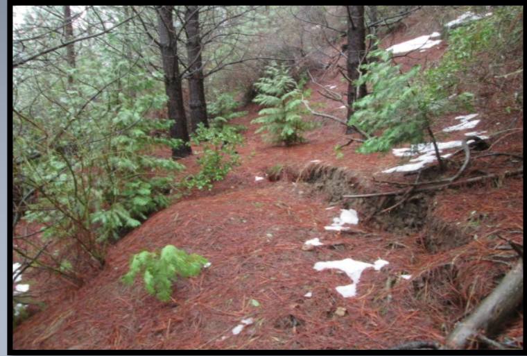
Soil cracking above canal flume 5
