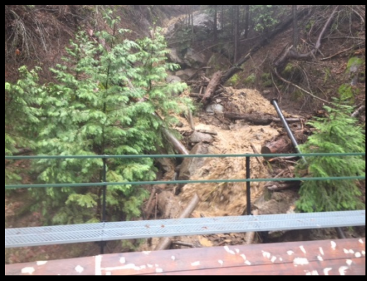
Flume 2A mud rock and tree removal 2/10/17
