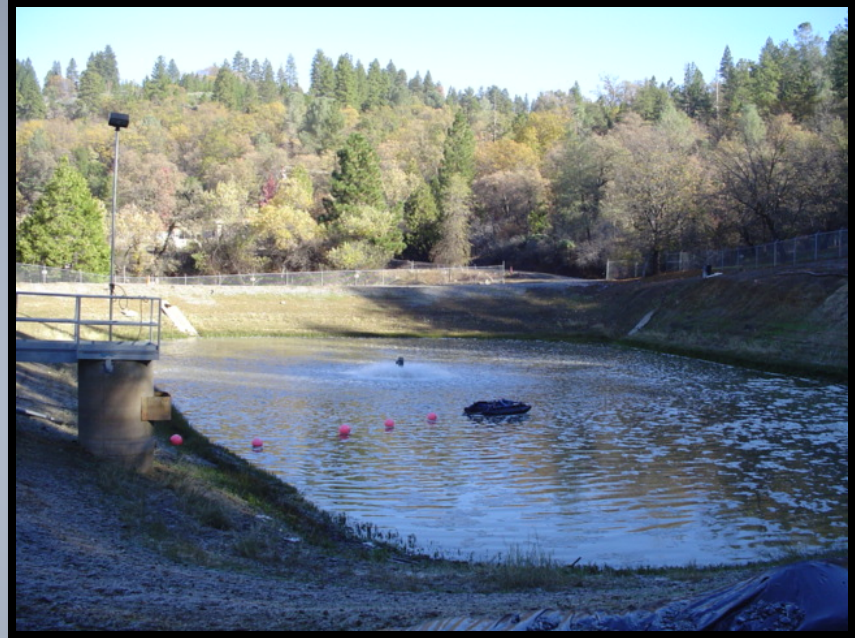
Camino Heights open pond treatment system
