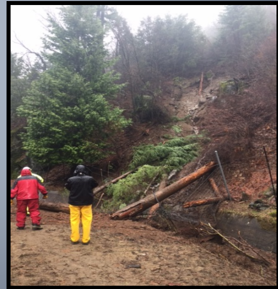
Crews remove debris and trees
