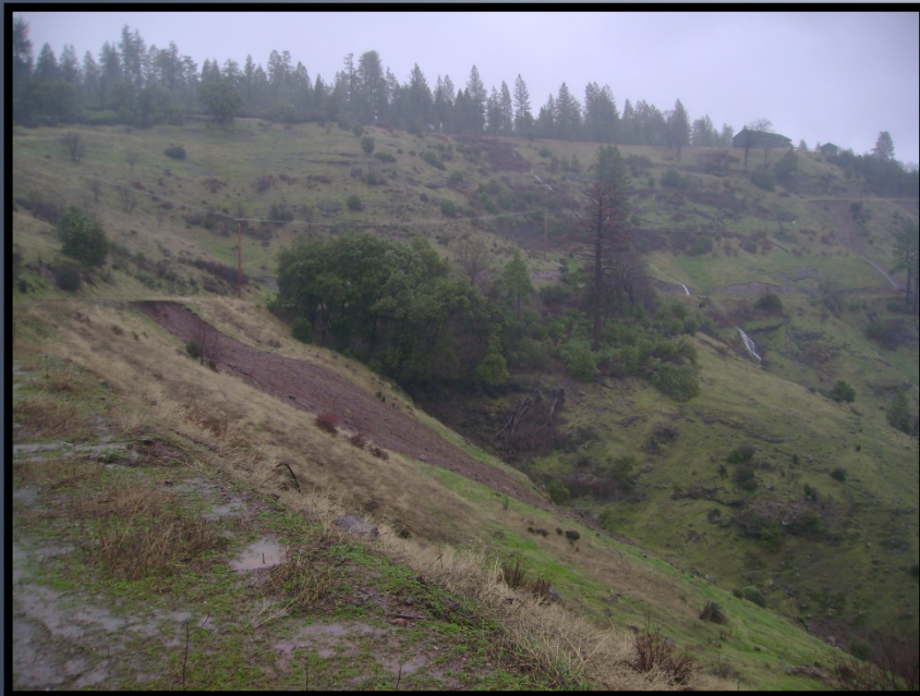
Transmission main is in the benched area
