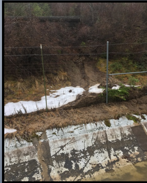
Flume 6 slide above canal 2/8/17
