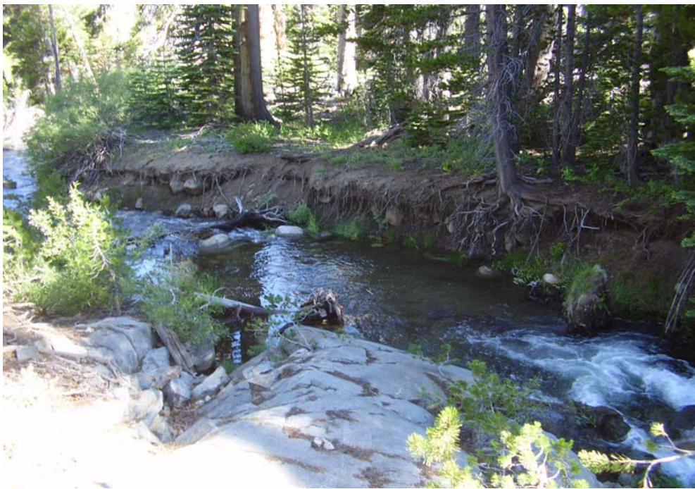
Figure 2-7 Upper Erosion Site right bank, with sloping bedrock on left bank
