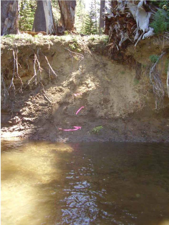
Erosion pins A, B, C (arranged vertically on left bank) installed just prior to the 58 cfs release. No photo available for post-flow release.
