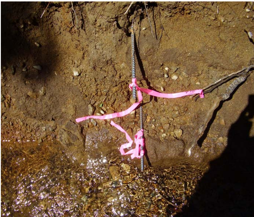
Approximately .5 ft bank retreat for both pins after 24 cfs release
