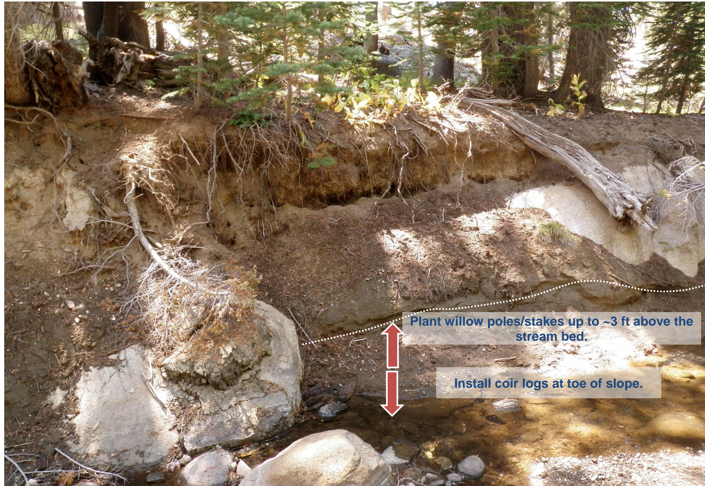
Figure 6b Upper Site – Treatment Area U-6: LB 2+46-1+39 (Photo 2 of 2)
