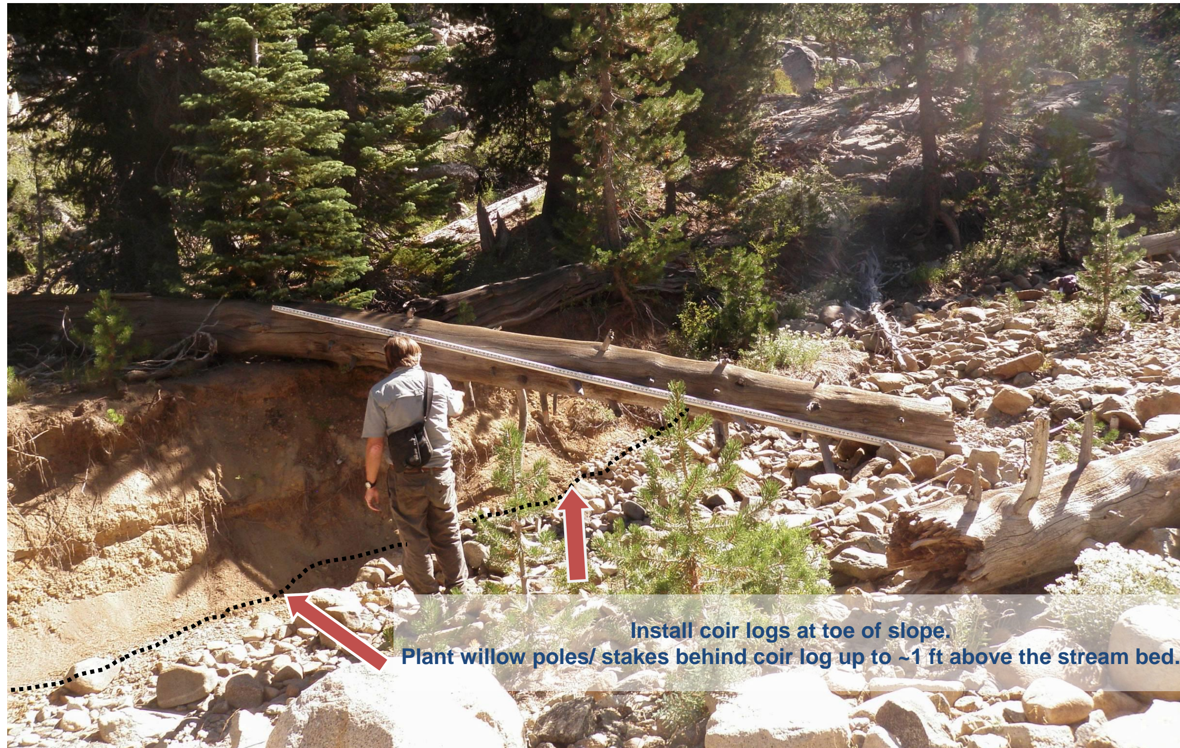
Figure 9a Lower Site – Treatment Area L-1: RB 8+48 to 7+74 (Photo 1 of 2)
