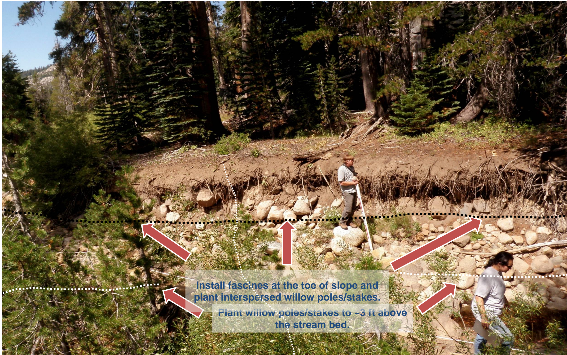
Figure 8 Upper Site – Treatment Area U-8: RB 0+64 to 0+01
