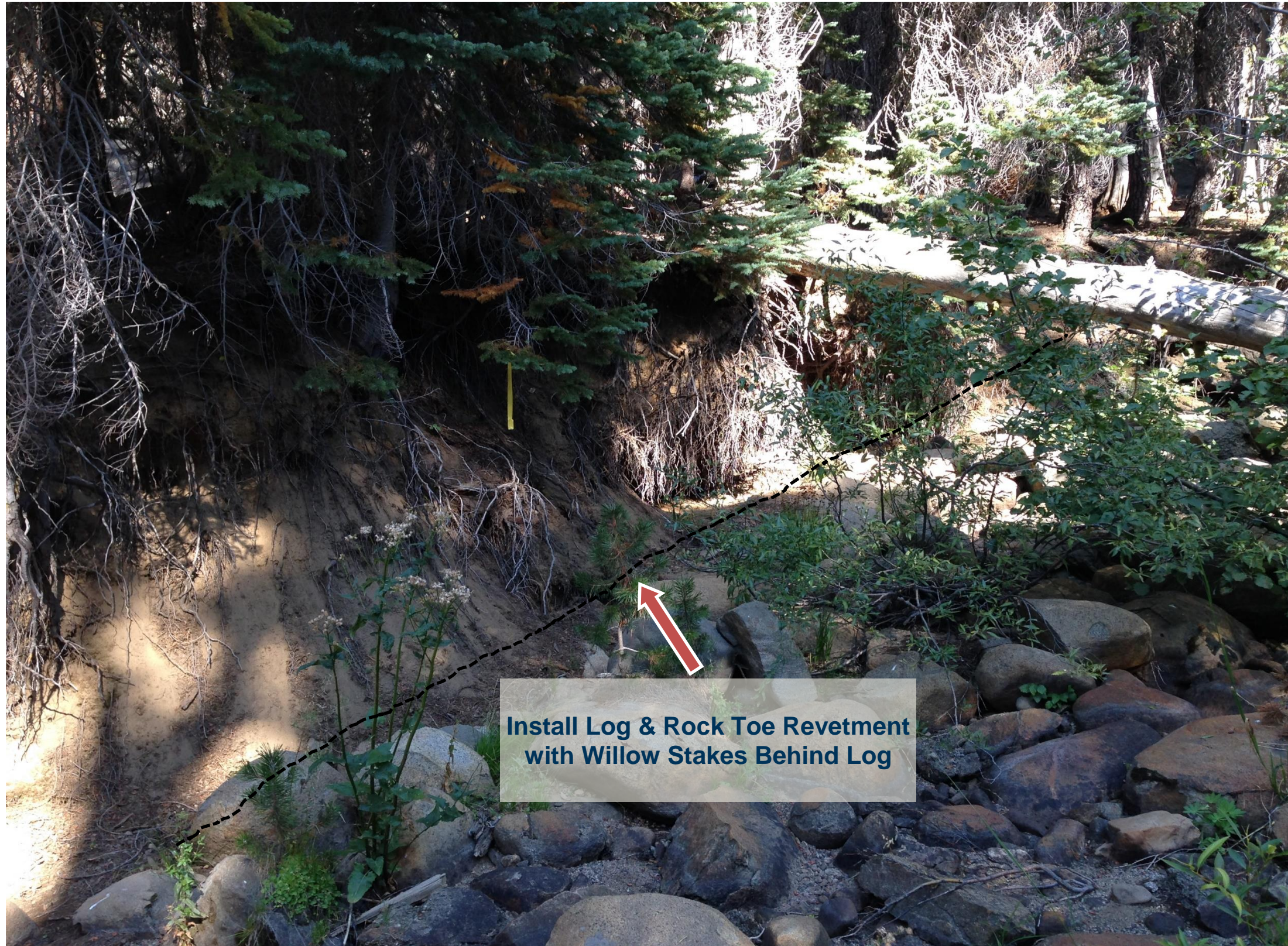
Figure 3 Upper Site - Treatment Area U-3: 2+45 to 3+30
