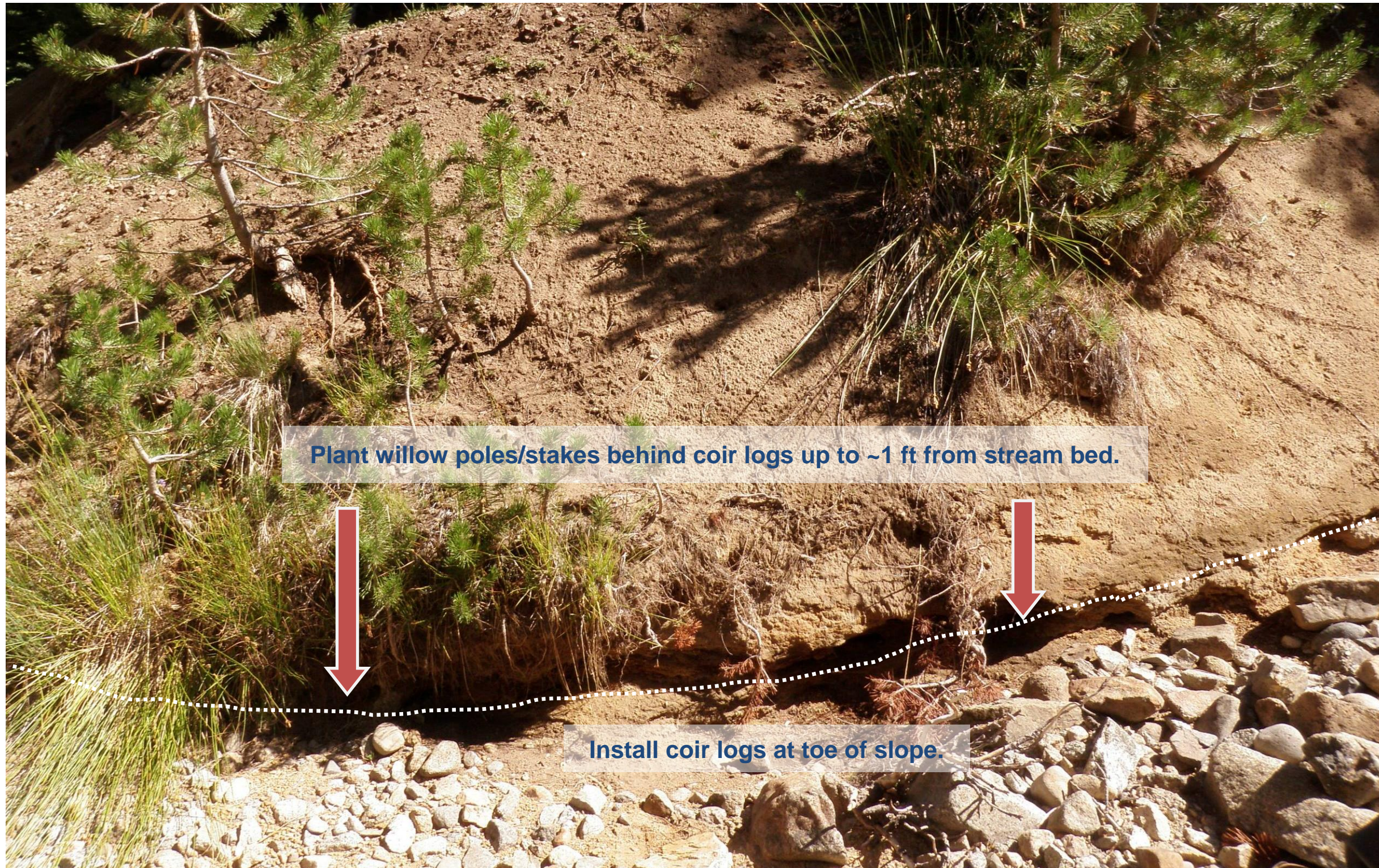
Figure 10 Lower Site – Treatment Area L-3: RB 7+38 to 7+02
