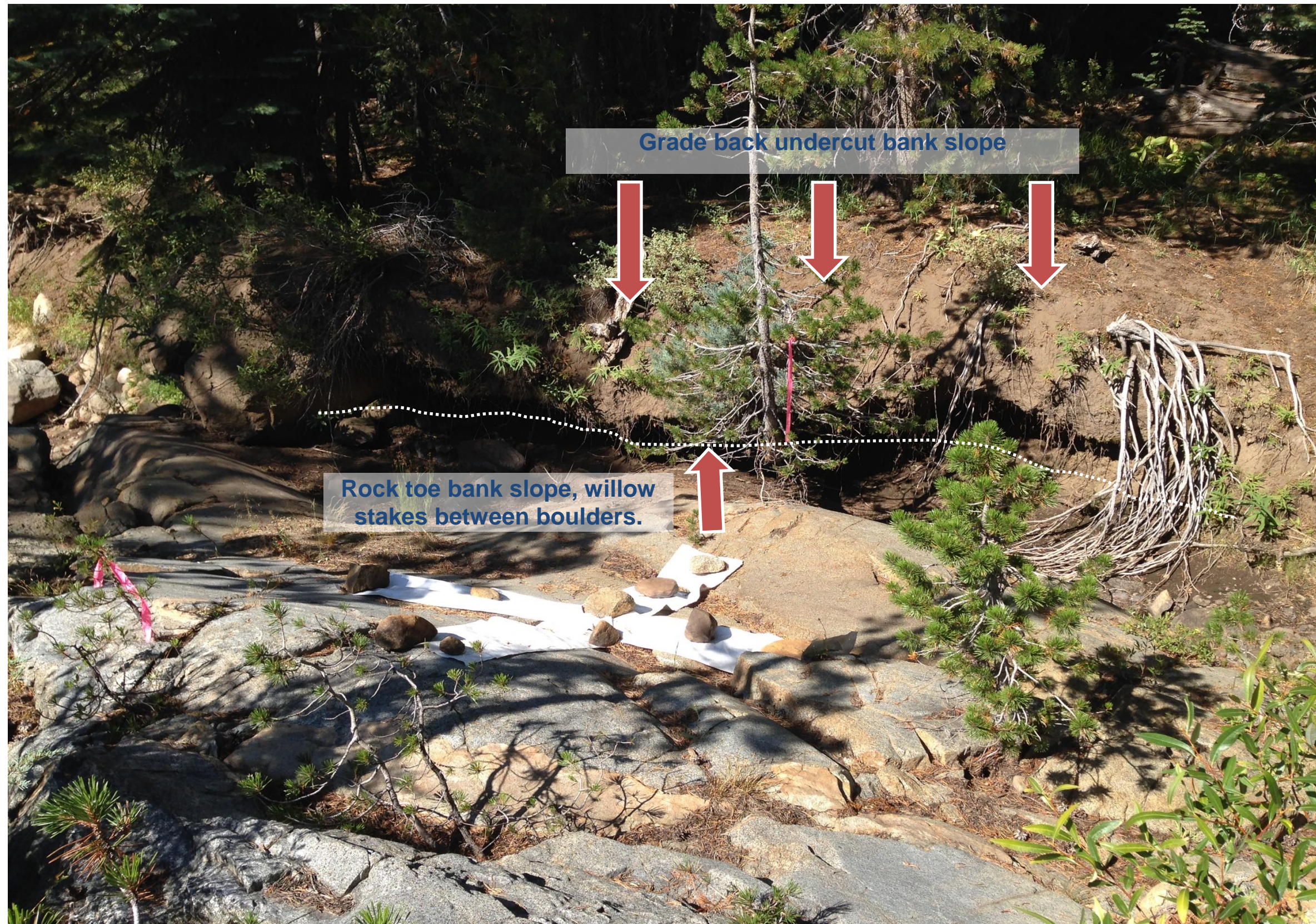
Figure 7. Upper Site – Treatment Area U-7: RB 0+60 to 1+08
