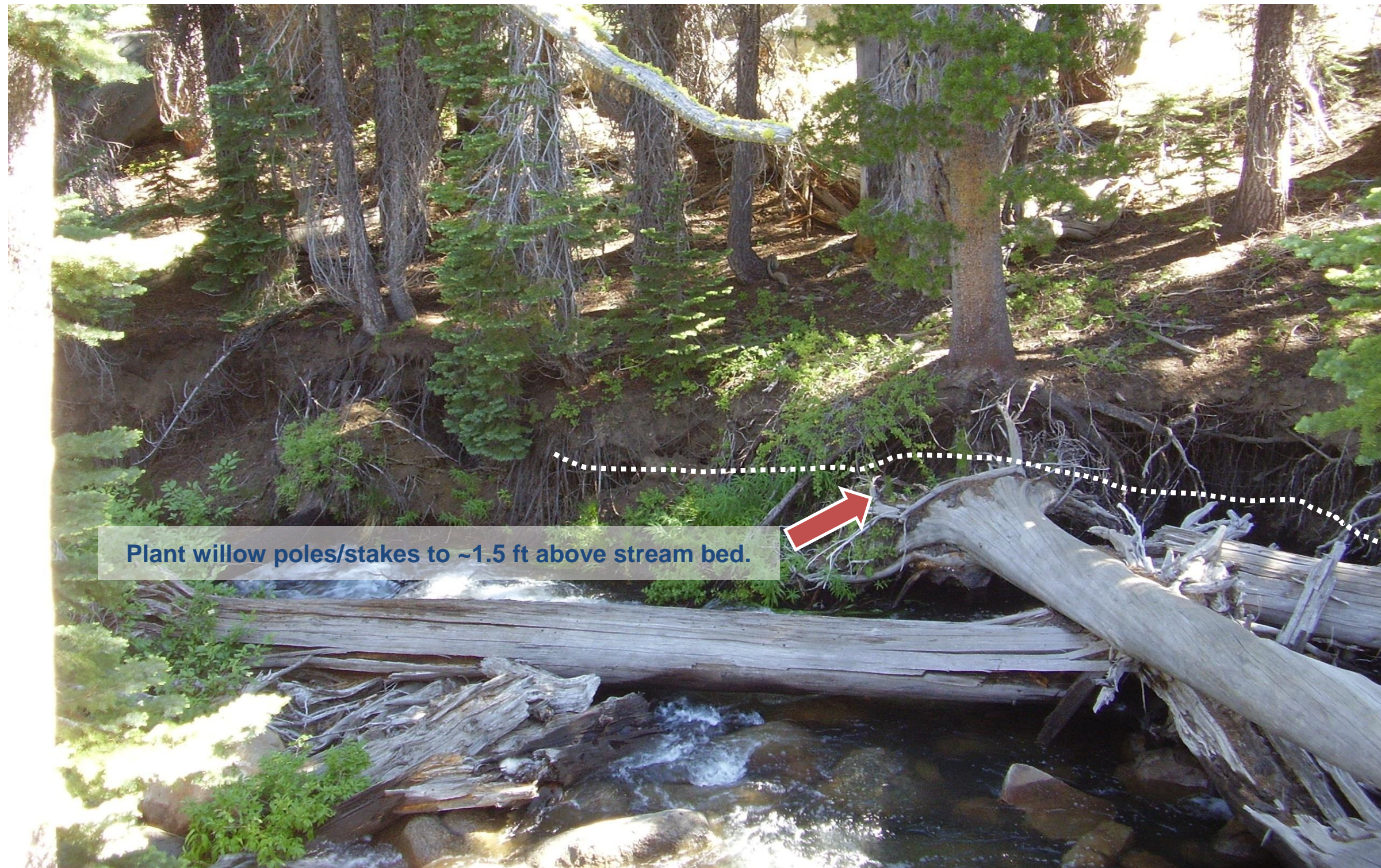
Figure 2 Upper Site – Treatment Area U-2: RB 3+57 to 3+17
