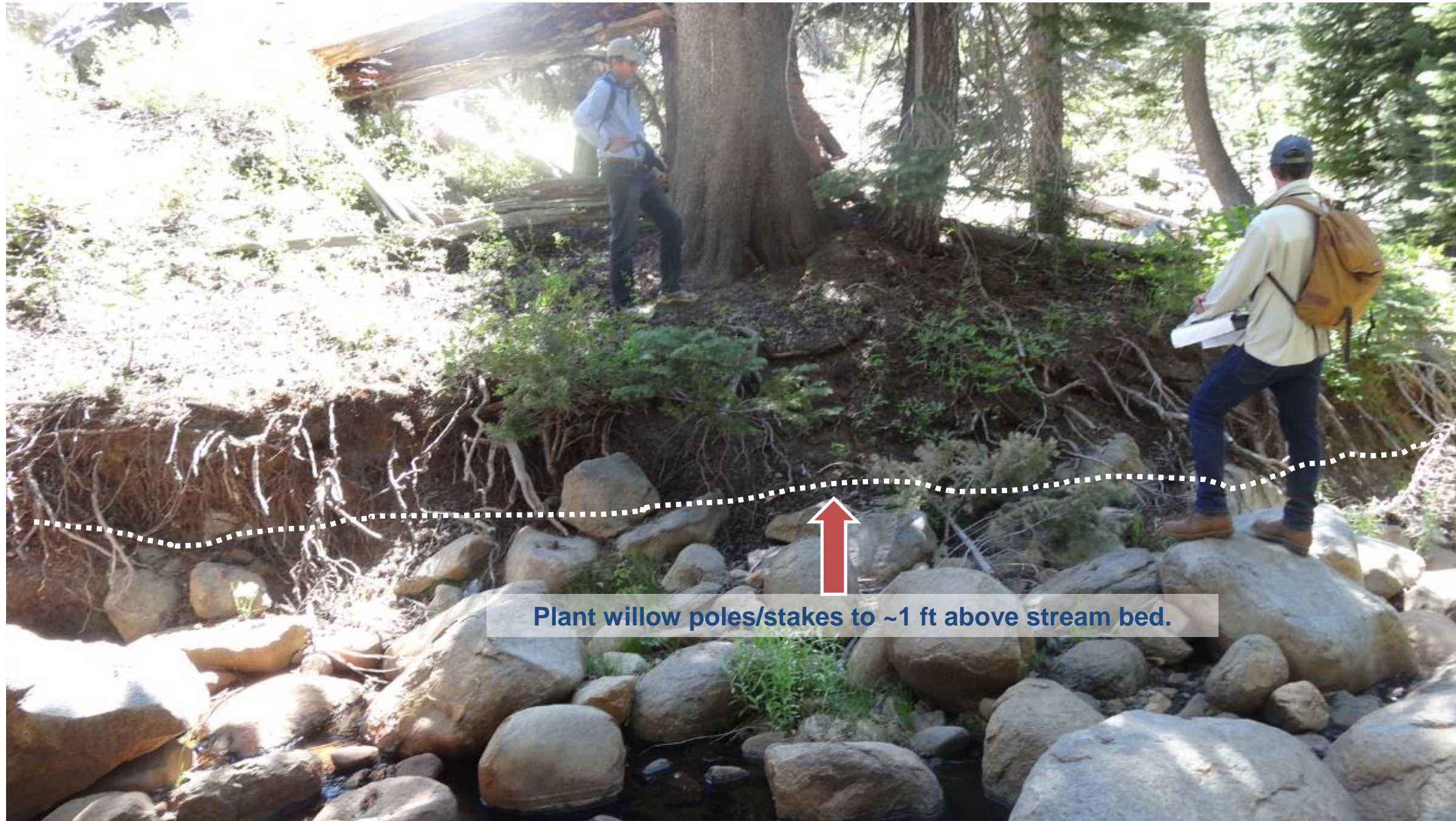
Figure 1 Upper Site – Treatment Area U-1: LB 3+55 to 3+25
