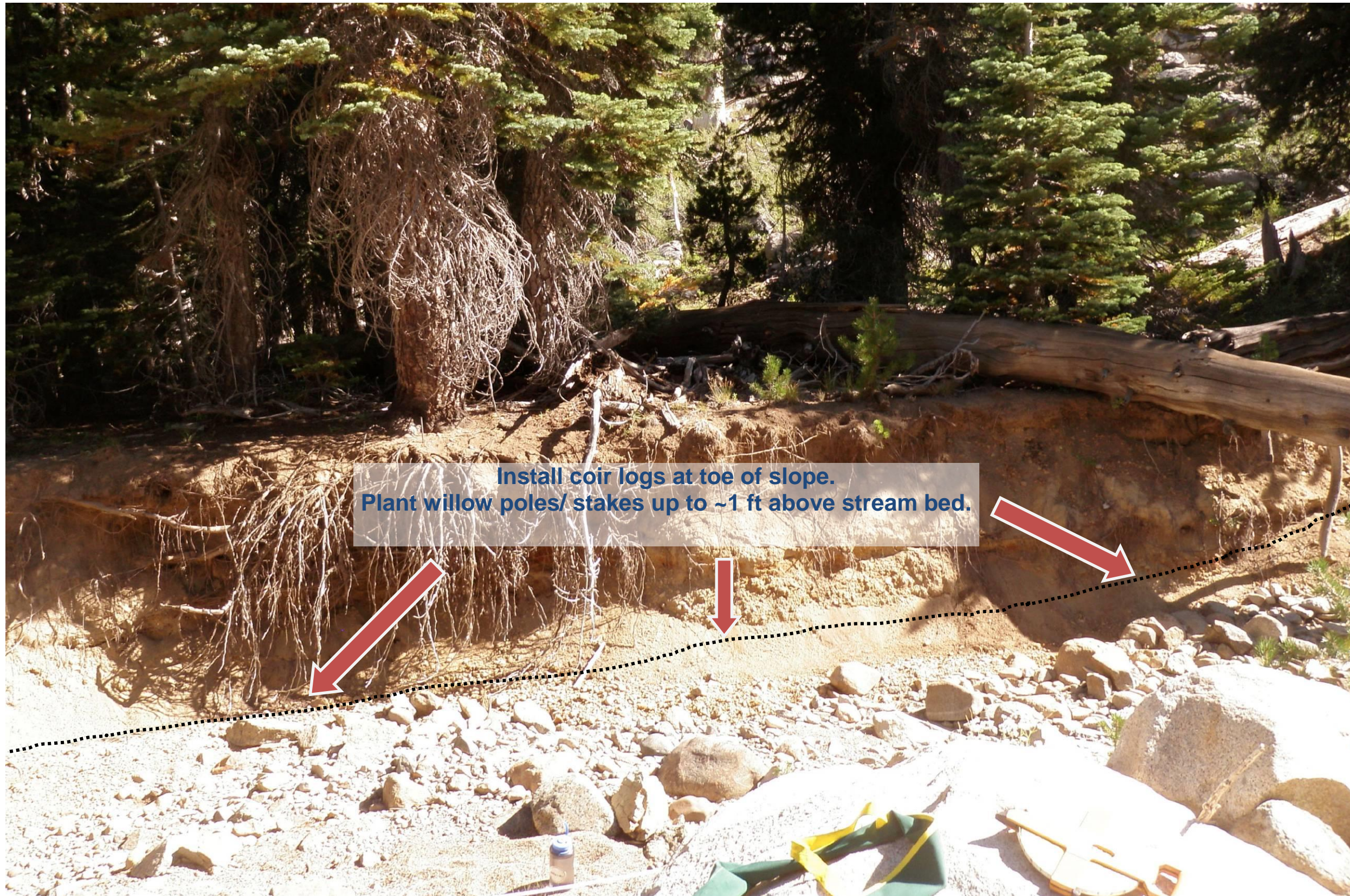
Figure 9b Lower Site – Treatment Area L-1: RB 8+48 to 7+74 (Photo 2 of 2)
