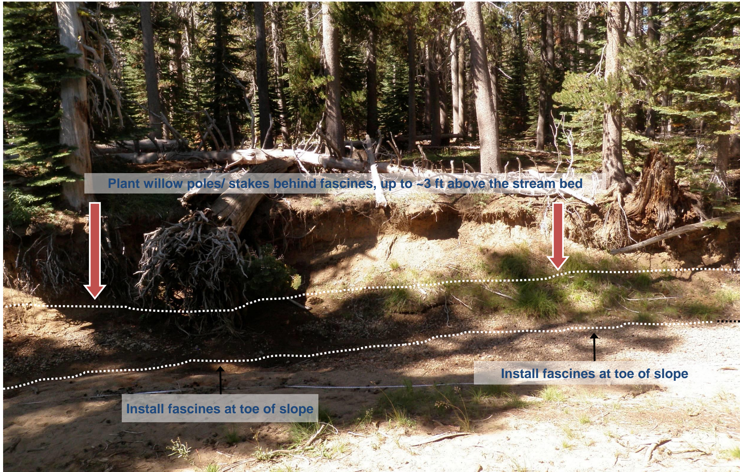
Figure 14d Lower Site - Treatment Area L-7: LB 5+20 to 4+13 (Photo 4 of 4)
